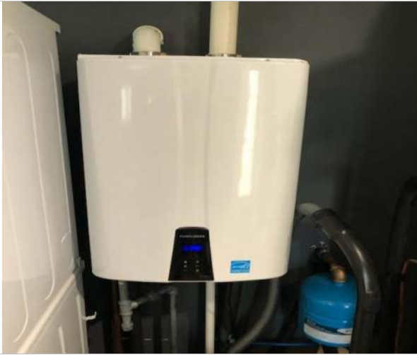
11. Tankless hot water heater
