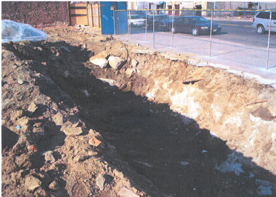
4. Grave of USTs after removal, E. 161 st Street in background
