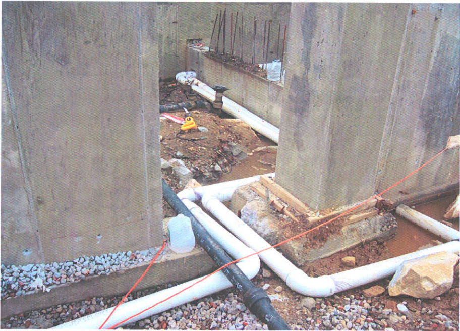
19. VES in basement area
