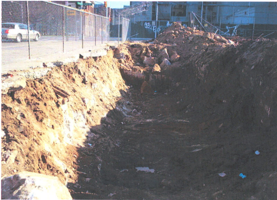
5. Grave of USTs, looking southeast
