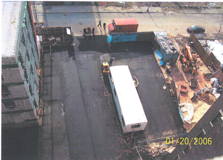
25. Asphalt-paved parking area (E. 160 th Street pictured)
