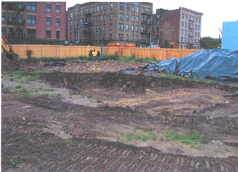
7. Area of pesticide-contaminated fill material (foreground), and covered, stockpiled material (background), looking south
