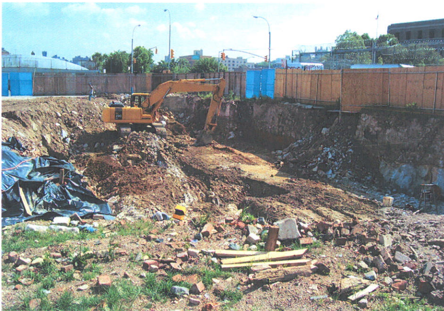
14. Basement area, near completion, looking east
