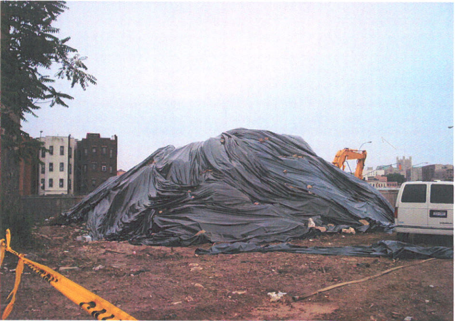
16. Covered, stockpiled fill material, looking east
