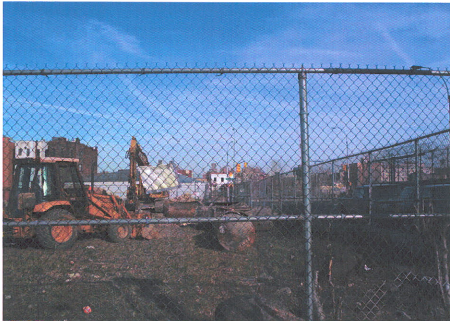
6. UST removal activities (taken from E. 160 th Street)
