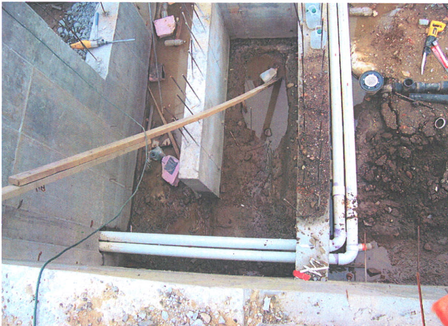
18. VES in basement area
