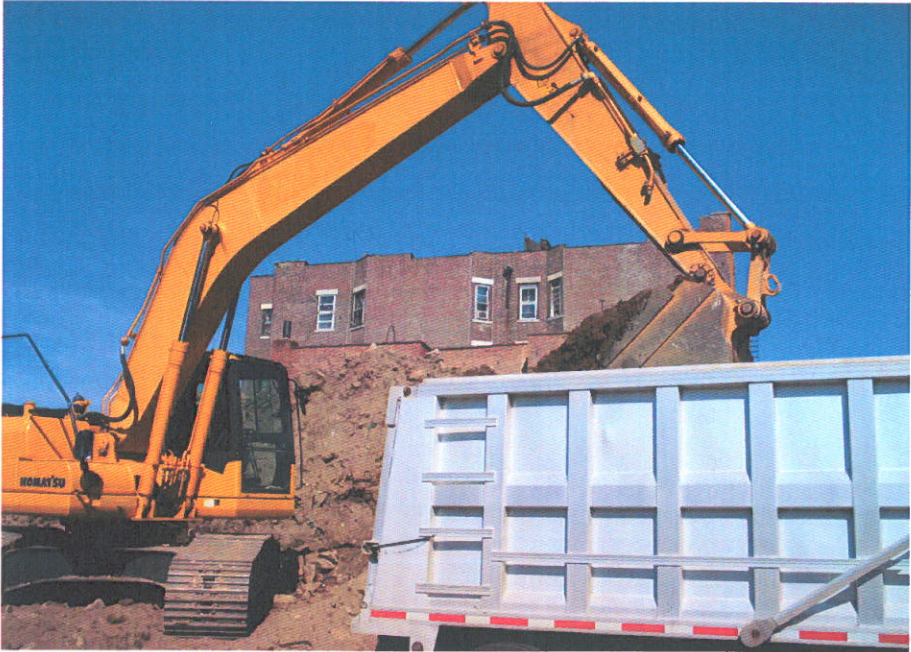
15. Removal of fill material
