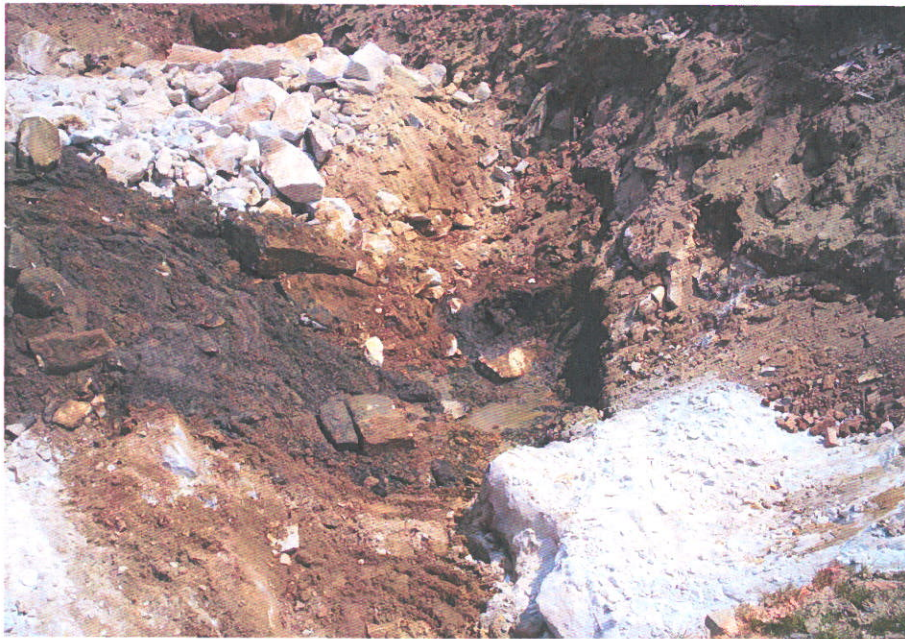
13. Stained soil in basement area
