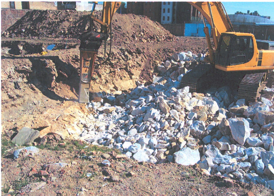
12. Breaking of bedrock in basement area, looking northeast
