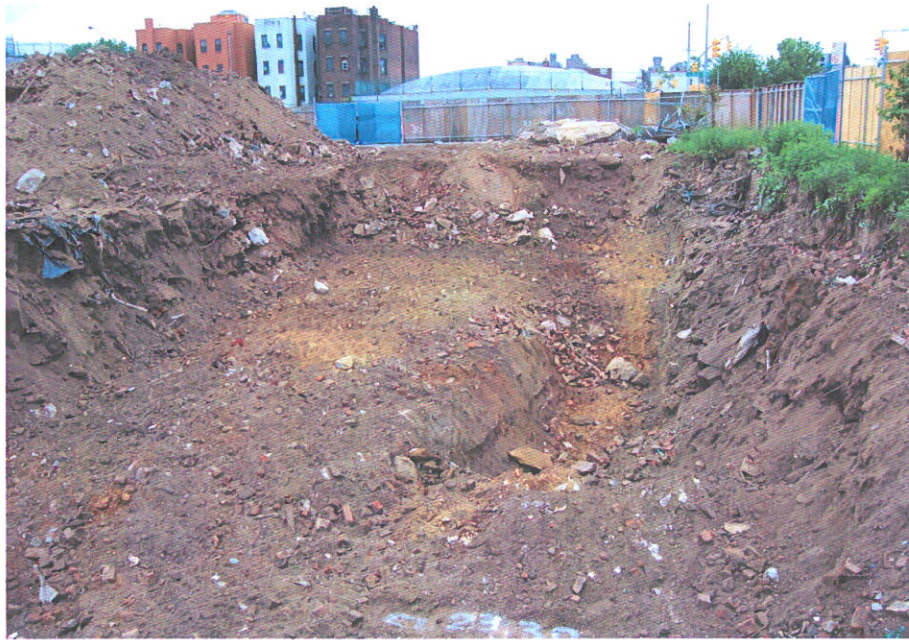
9. Basement area at bedrock interface (elevation: 23.30'), looking northeast
