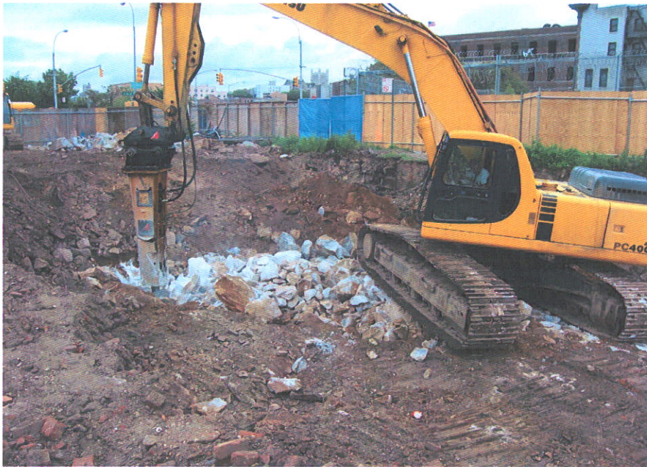
11. Breaking of bedrock in basement area, looking east
