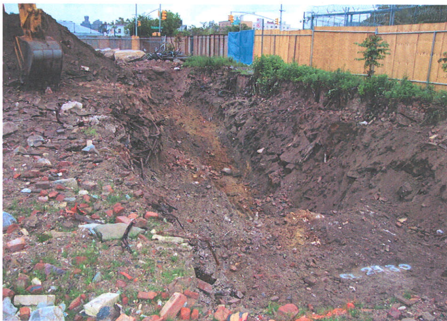
8. Early stage soil removal of initial excavation (basement) area, looking east
