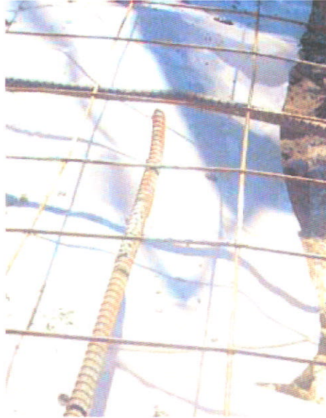
27. Vapor barrier installation beneath the slab
