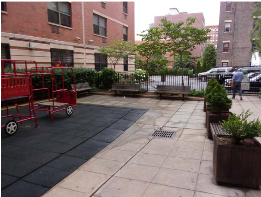
2. View of courtyard barrier layer
