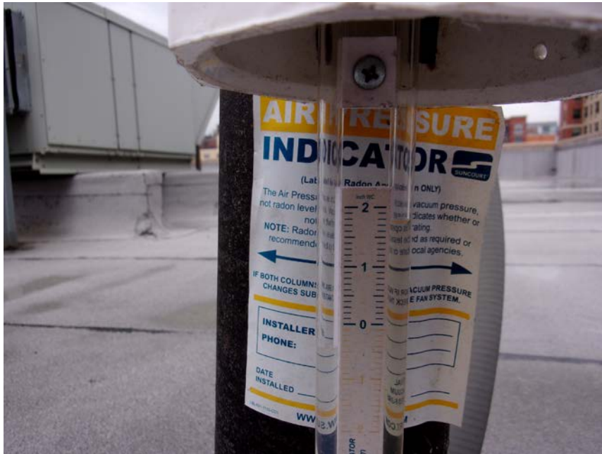
7. View of U-manometer corresponding to VP-3
