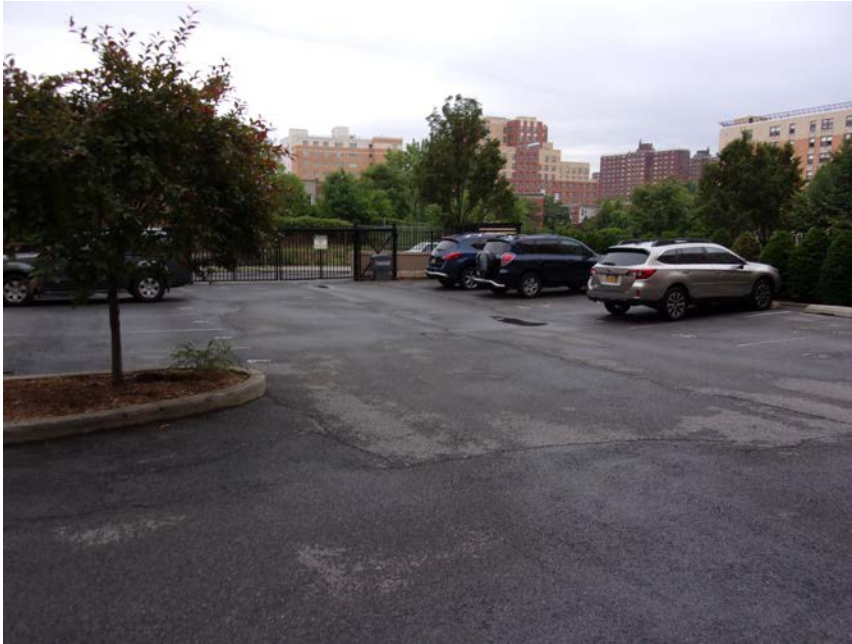
View of paved parking barrier layer
