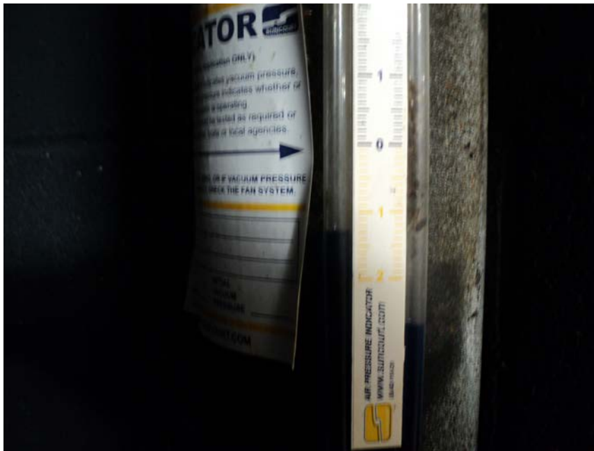
13. U-manometer located at vertical pipe VP-1 on December 2, 2016.
