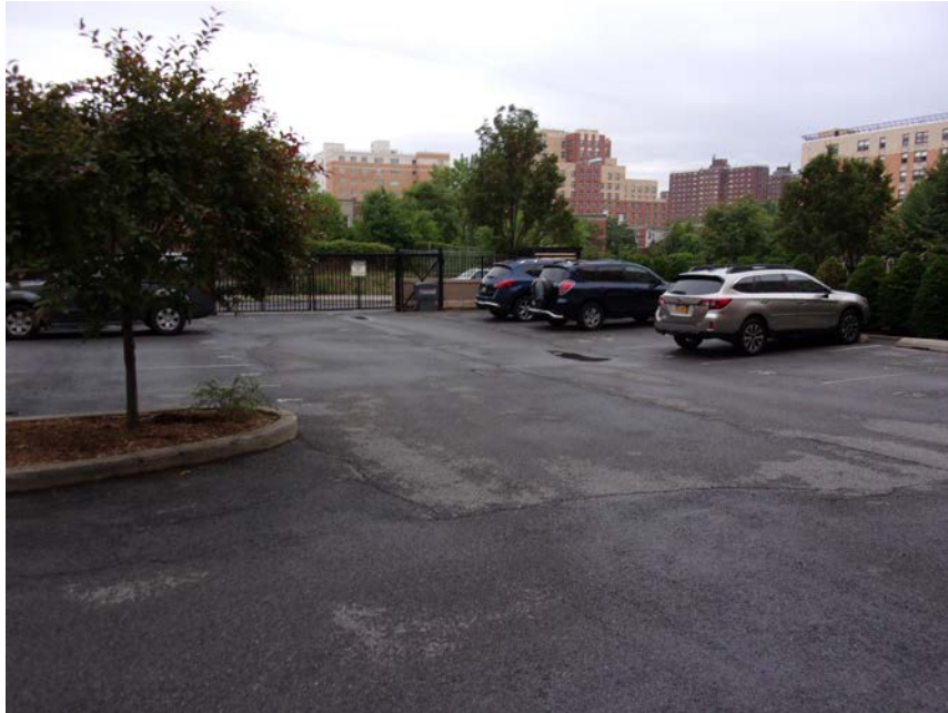
View of paved parking barrier layer in June 2016.
