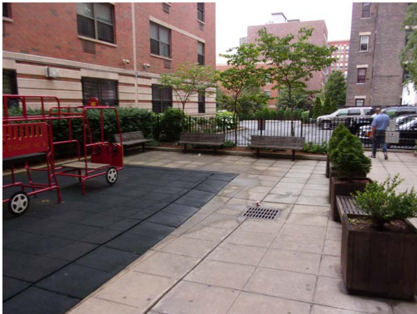
2. View of courtyard barrier layer in June 2016.
