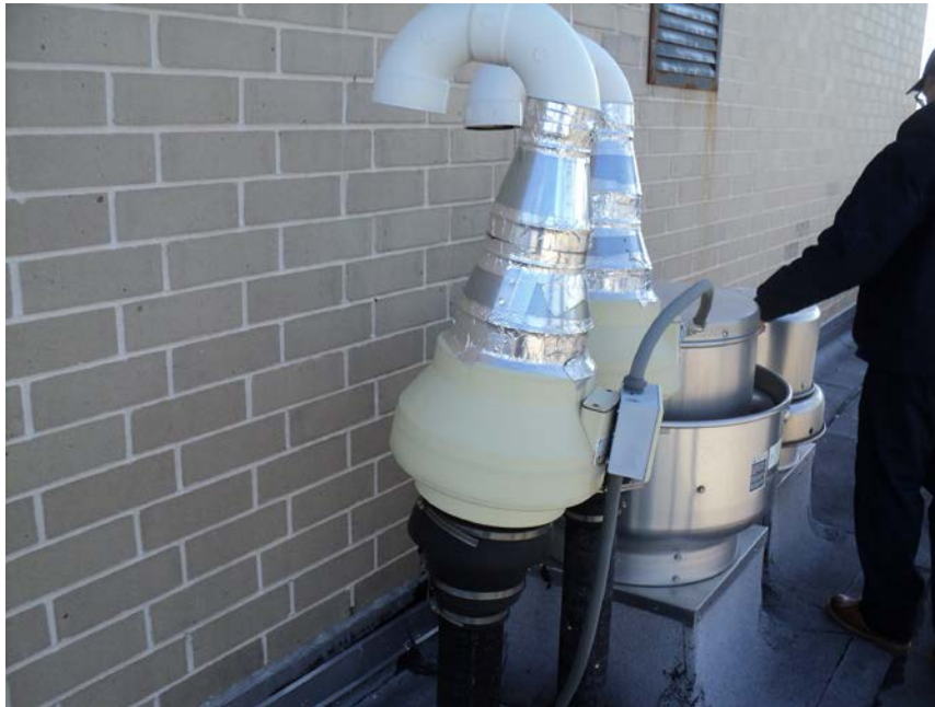
15. View of VES fans connected to VP-1 and VP-2, located at the roof level, on December 2, 2016.
