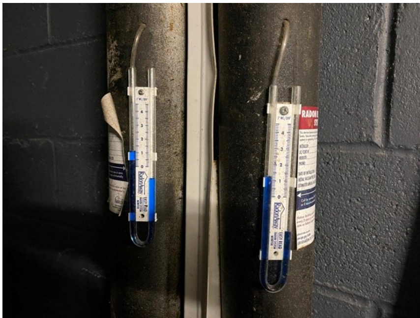
4. U-manometers corresponding to VP-1 (left) and VP-2 (right), both displaying negative pressure readings
