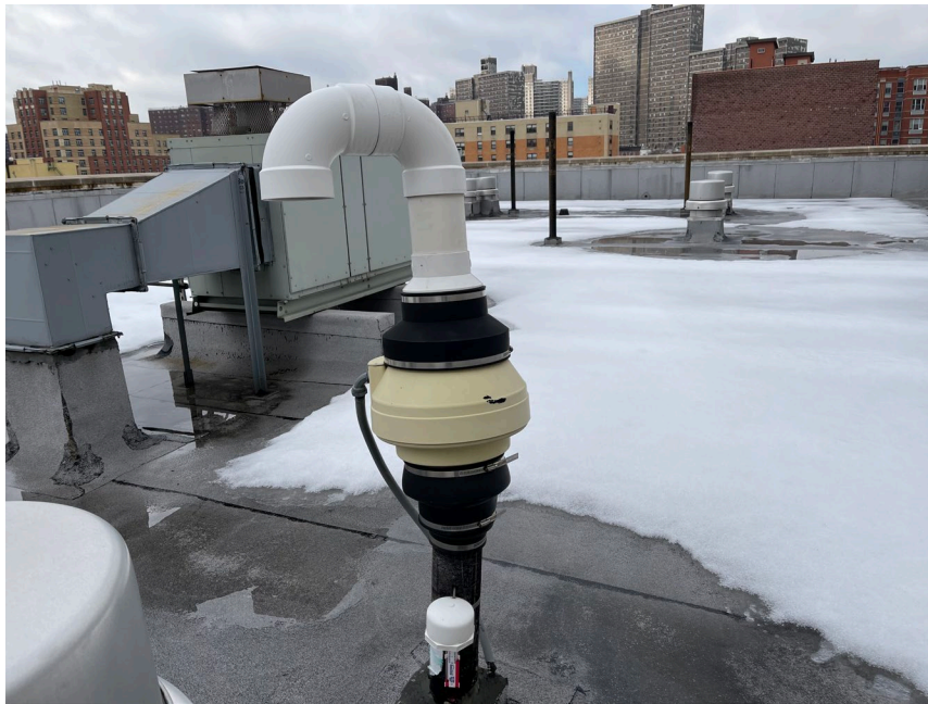
7. VES fan connected to VP-3, located on southern roof
