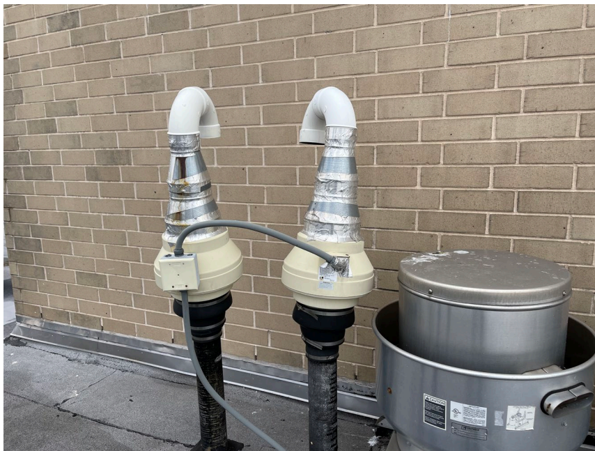
8. VES fans connected to VP-1 and VP-2, located on roof
