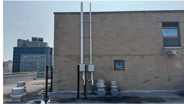
6. VES fans connected to VP-1 and VP-2, located on roof
