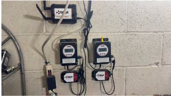
5. Audible alarms and visual gauges for VP-1 (left) and VP-2 (right) displaying negative pressure readings
