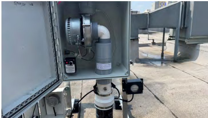
7. Gauge corresponding to VP-3 displaying negative pressure reading
