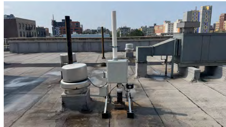
8. VES fan connected to VP-3, located on southern roof
