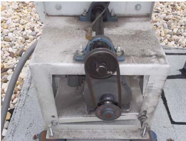
Photo 3: View of typical fan belt assembly (F-5).
