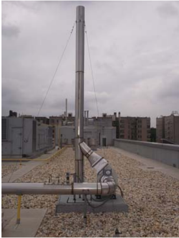
Photo 1: View of typical SSDS roof fan unit (F-5).
