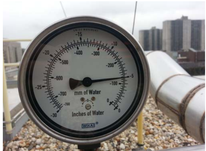
Photo 4: View of typical vacuum gauge associated with SSDS fan units (EF-4).
