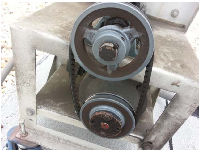
Photo 5: View of typical SSDS fan belt (EF-5).
