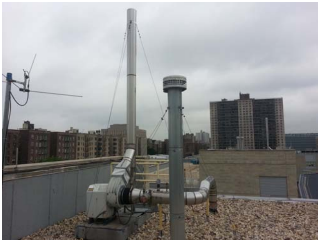
Photo 3: View of typical SSDS roof fan unit (EF-4).
