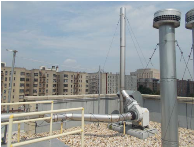
Photo 3: View of typical SSDS roof fan unit (EF-2).
