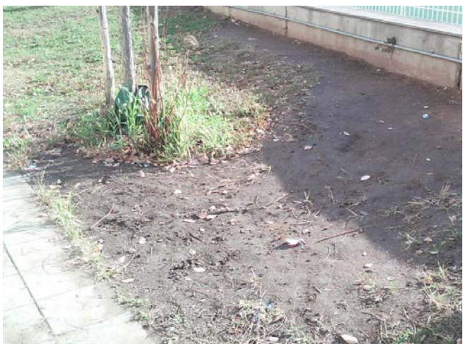
Photo 12: View repairs made to the soil erosion (4.5' x 2' x 2'') adjacent to the auditorium building.
