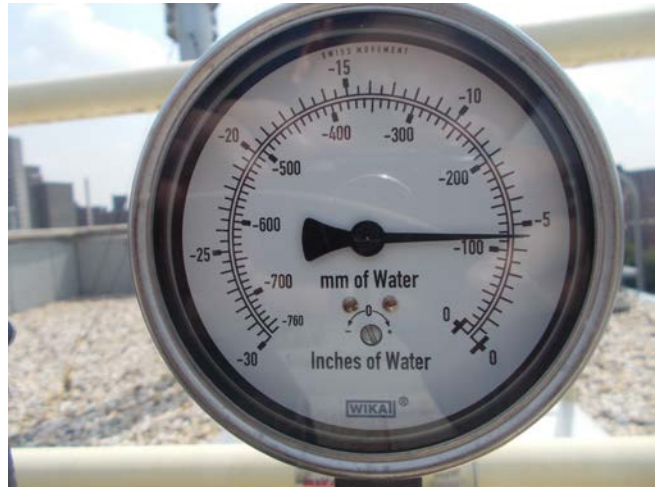
Photo 4: View of typical vacuum gauge associated with SSDS fan units (EF-2).
