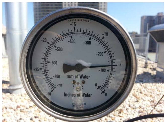
Photo 6: View of typical vacuum gauge associated with SSDS fan units (EF-1).
