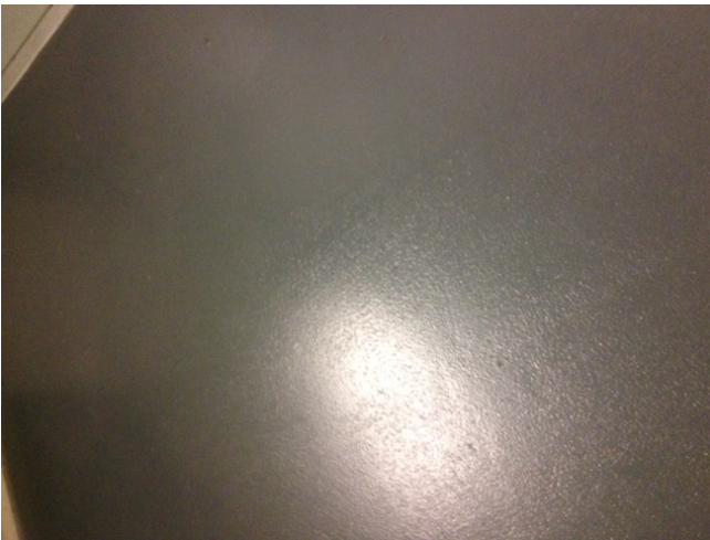
Photo 9: View of typical bare concrete floor in Stairwell H.
