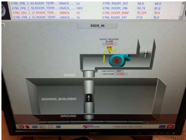
Photo 3: View of BMS incorrectly indicating an alarm on fan unit SSDS-6.
