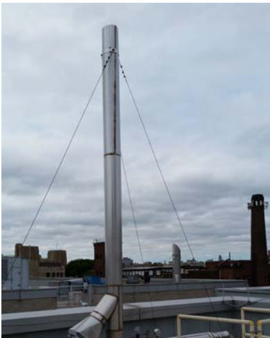
Photo 3: View of typical SSDS roof fan unit EF-2.
