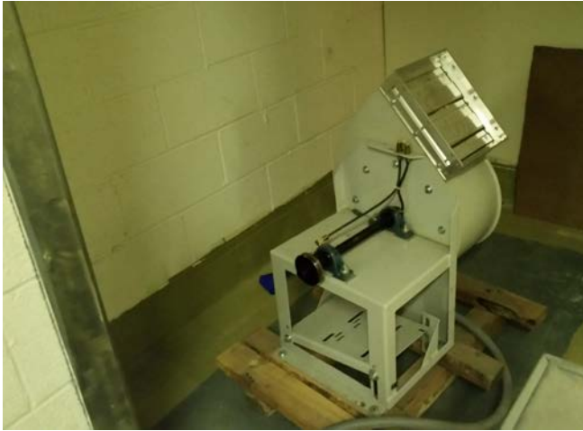
Photo 7: View of spare SSDS fan unit in Room B80.
