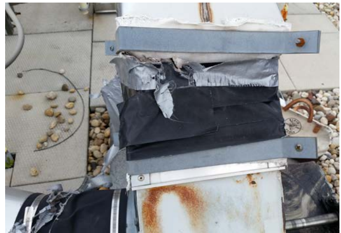
Photo 6: View of damaged flex joint cloth associated with SSDS fan unit EF-6.
