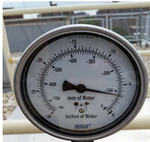
Photo 4: View of typical vacuum gauge associated with SSDS fan unit EF-2.
