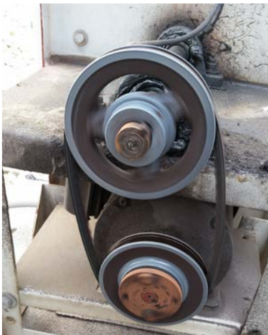
Photo 5: View of typical motor-fan assembly EF-2.
