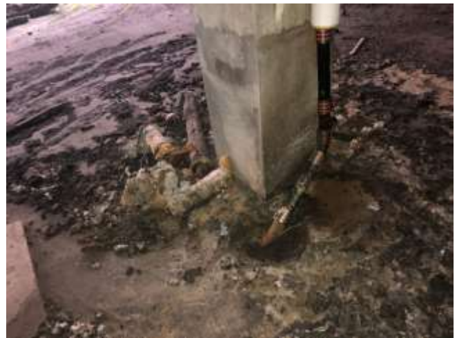
Photo 10: Damaged concrete around column on concrete cap area below P.S. 151X.
