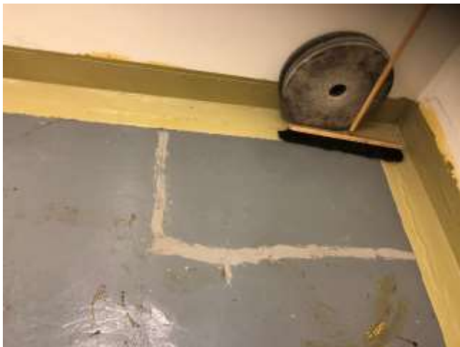
Photo 3: View of patched hairline cracks in Room C86.
