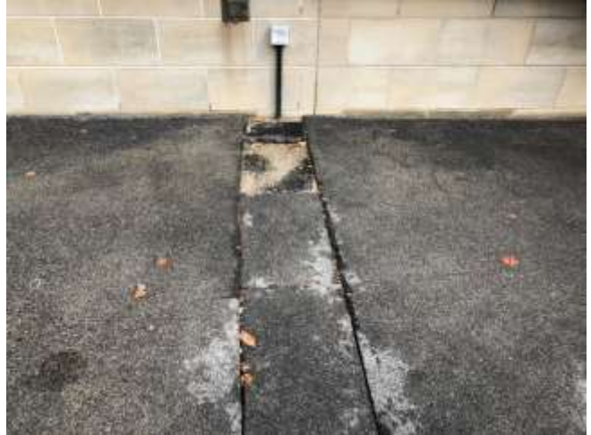
Photo 14: Area of damaged asphalt pavement south of Tower D reportedly due to a rerouted conduit line.
