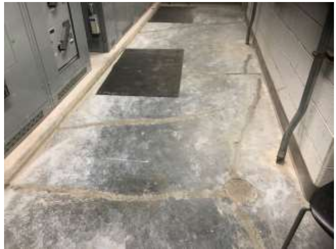
Photo 2: View of patched hairline cracks in Room C20.
