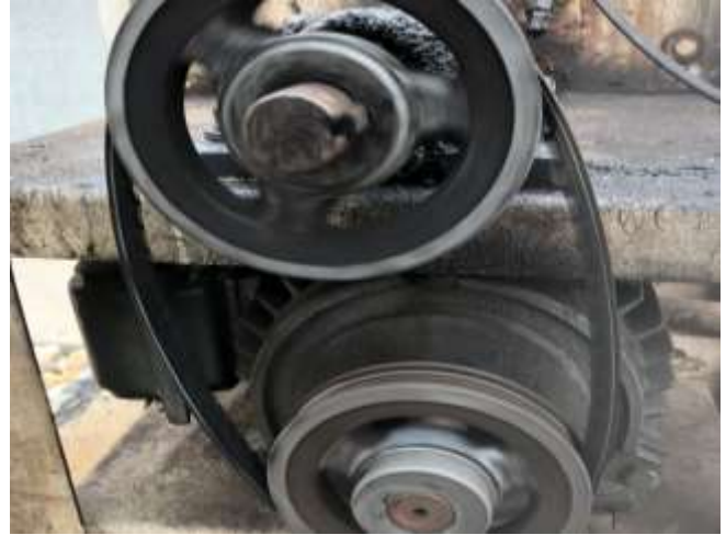
Photo 8: Loose belt observed on SSDS fan unit EF-6.
