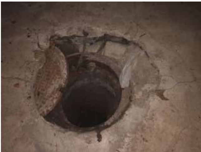
Photo 9: Damaged concrete around north manhole on concrete cap area below P.S. 151X.
