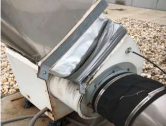
Photo 7: View of damaged flex joint cloth associated with SSDS fan unit EF-6.
