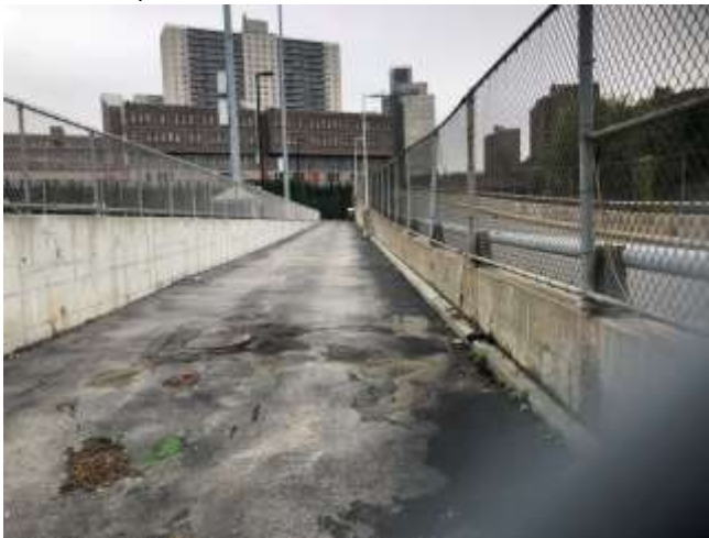
Photo 11: View of damage on the asphalt pavement at the fire lane exit gate.
