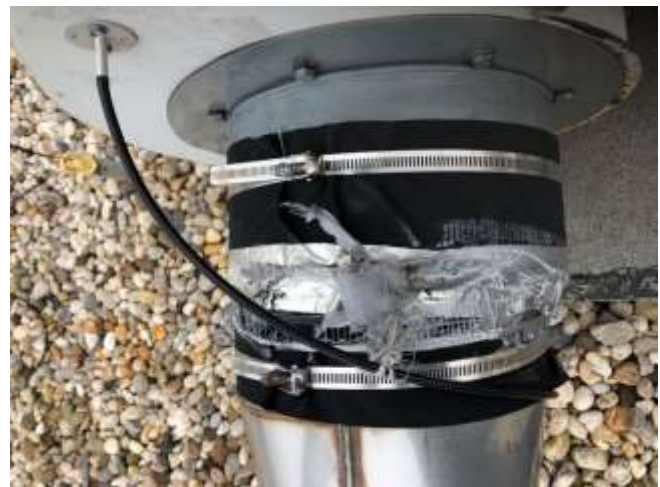
Photo 6: View of damaged flex joint cloth associated with SSDS fan unit EF-4.
