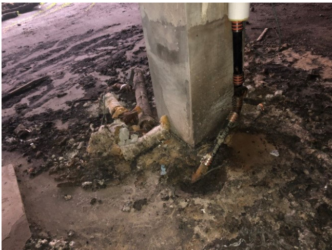
Photo 17: Damaged concrete around column on concrete cap area below P.S. 151X.
