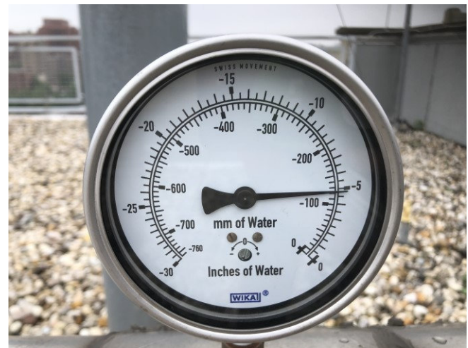
Photo 12: View of typical vacuum gauge associated with SSDS fan unit EF-4.
