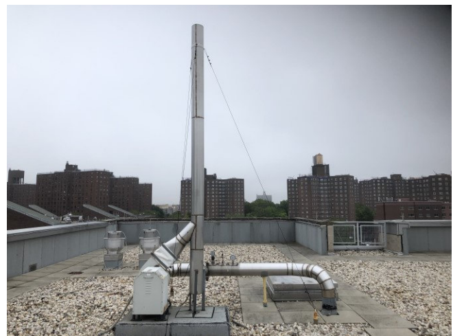
Photo 6: View of SSDS fan unit EF-5.
