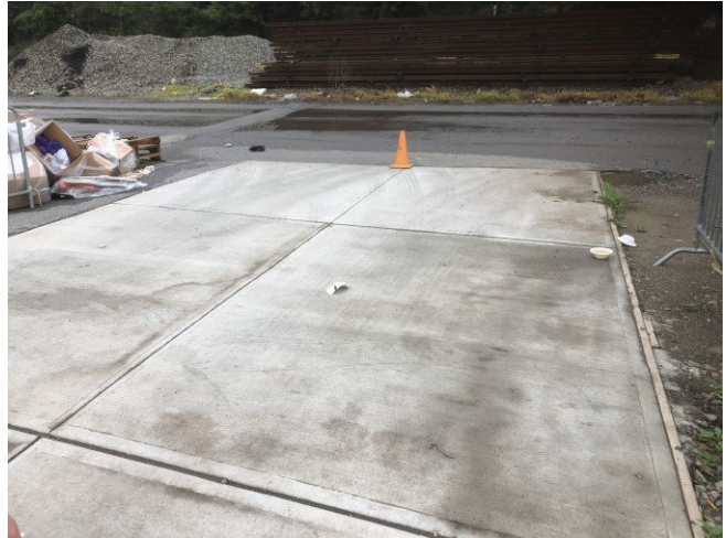
Photo 20: Repairs completed for compactor concrete pad.
