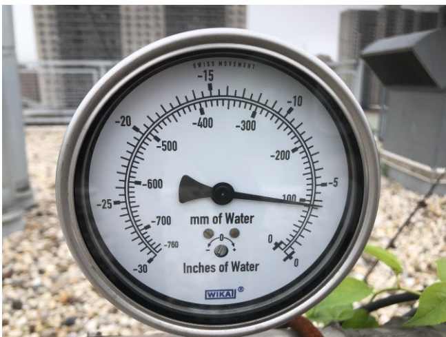
Photo 5: View of typical vacuum gauge associated with SSDS fan unit EF-1.
