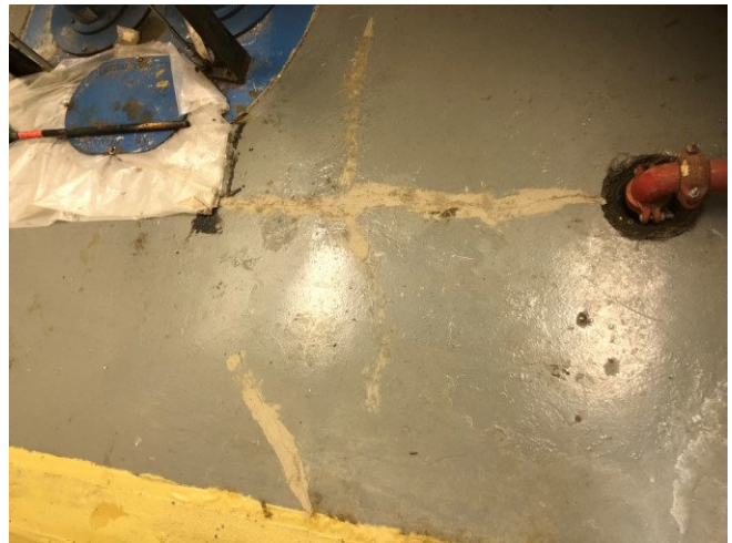
Photo 2: View of patched hairline cracks in Room C86.
