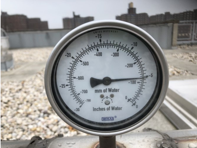
Photo 7: View of typical vacuum gauge associated with SSDS fan unit EF-5.
