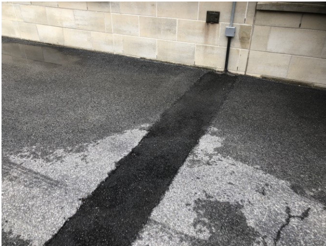
Photo 19: Repairs completed for compactor concrete pad.
