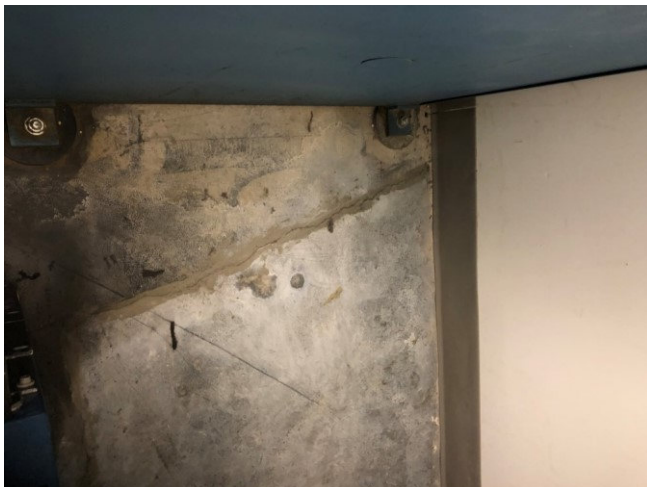
Photo 3: View of patched hairline cracks in Room C80J.
