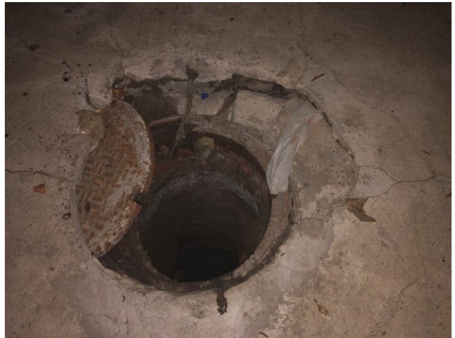
Photo 16: Damaged concrete around north manhole on concrete cap area below P.S. 151X.
