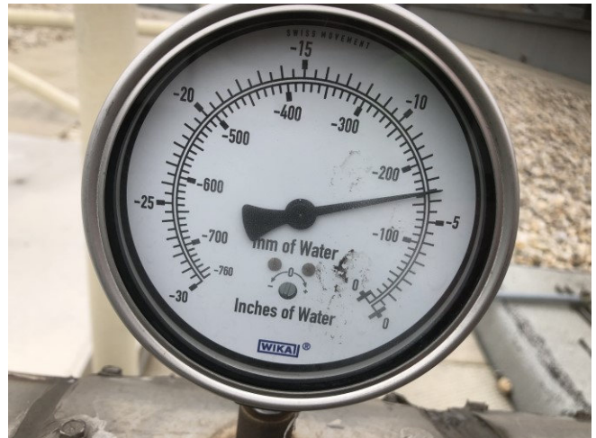
Photo 10: View of typical vacuum gauge associated with SSDS fan unit EF-6.
