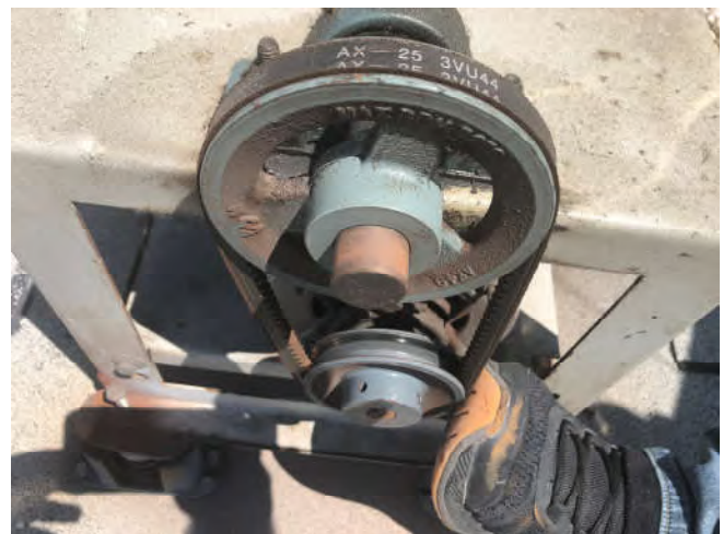
Photo 6: View of typical SSDS fan/motor assembly (EF-1).
