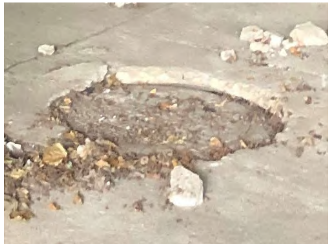
Photo 10: View of repaired patch around south manhole on concrete cap under P.S. 151X with minor chipping.
