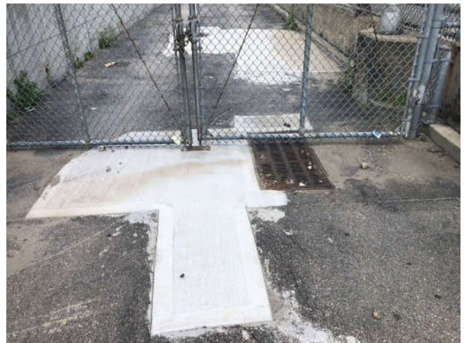
Photo 12: Area of concrete patch around adjacent to drain inlet at the fire lane exit gate.
