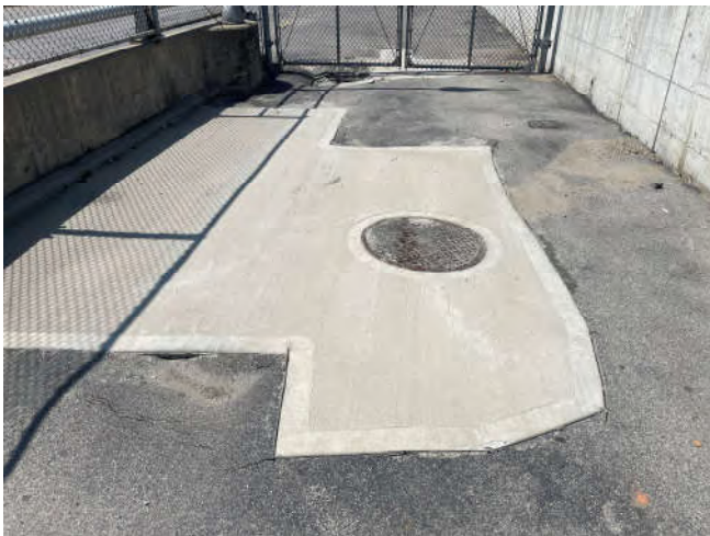
Photo 11: Area of concrete patch around manhole at the fire lane exit gate
