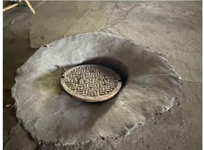
Photo 8: View of repaired patch around north manhole on concrete cap under P.S. 151X.
