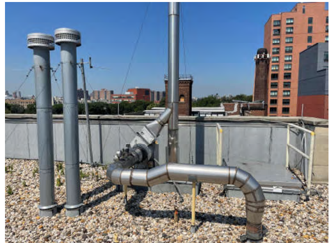
Photo 4: View of typical SSDS fan unit (EF-4).
