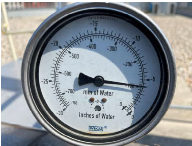
Photo 5: View of typical SSDS vacuum gauge (EF-6).
