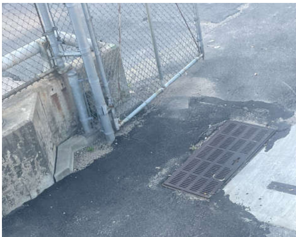
Photo 11: Area of asphalt patch around storm drain at the fire lane exit gate
