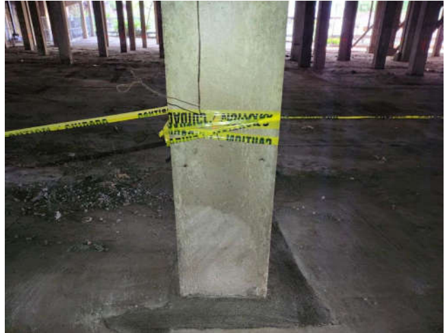
Photo 8: View of repaired patch around Column 193.
