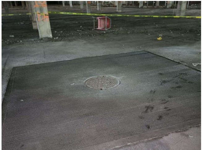
Photo 10: View of repaired patch around Manhole 10.
