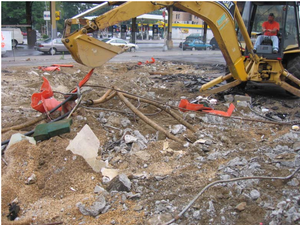
Dispenser 2 and Associated Piping Being Removed
