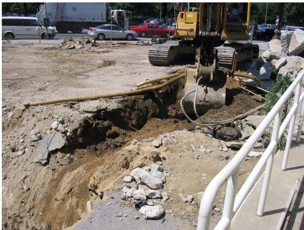
Dispenser Piping Leading to UST Excavation Being Removed
