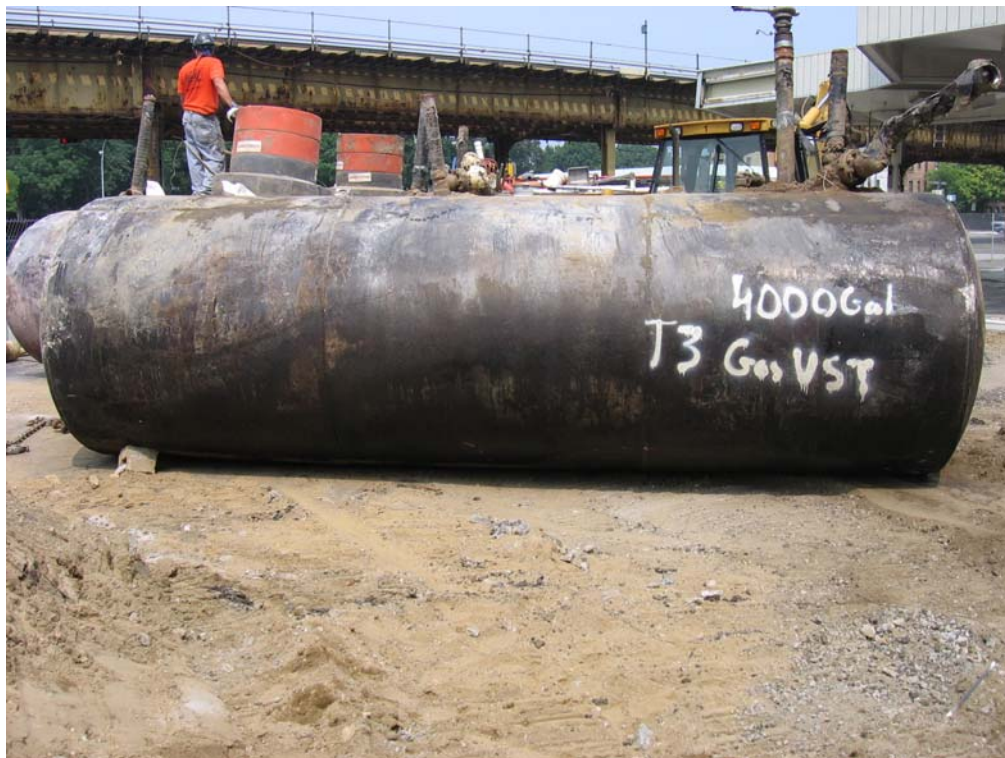
Tank3 – 4,000 gallon Gasoline UST
