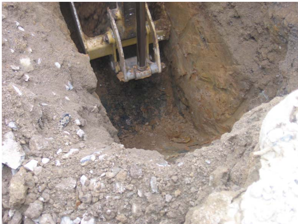
Bedrock Bottom of Former Waste Oil UST Excavation
