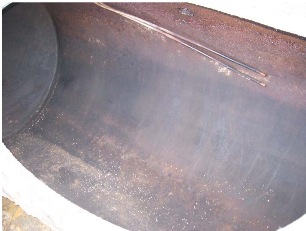
Tank4 – Interior of 550 gallon Fuel Oil UST
