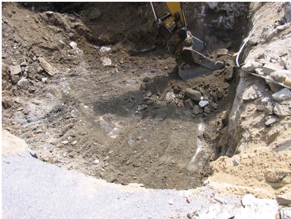
Bedrock Bottom of UST Excavation
