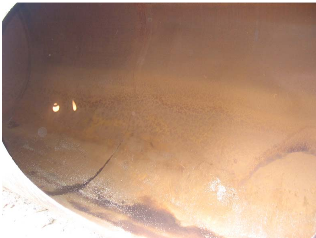
Tank2 – Interior of 4,000 gallon Gasoline UST
