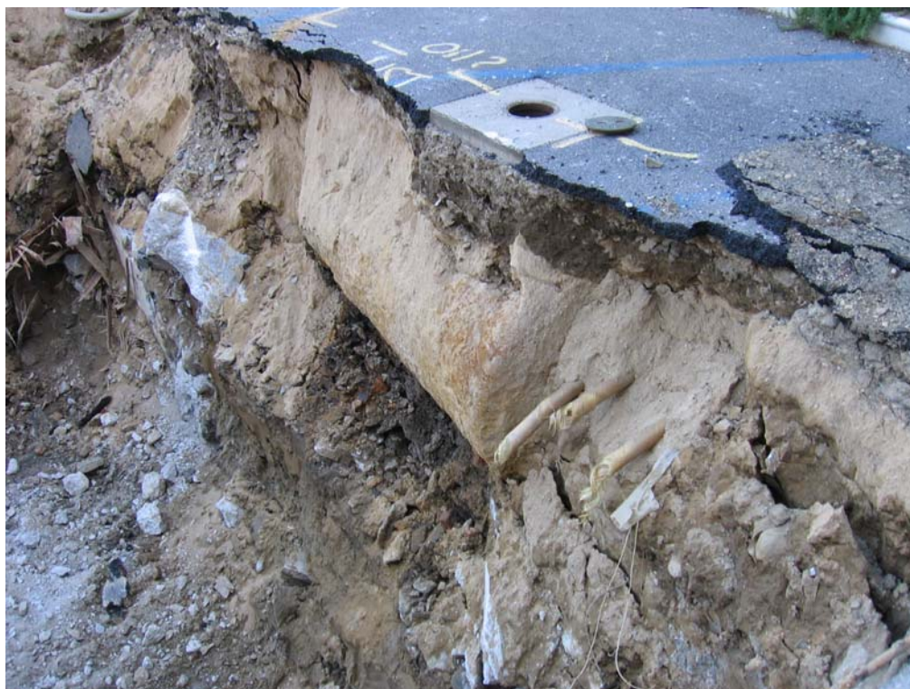
Tank4 – 550 gallon Fuel Oil UST
