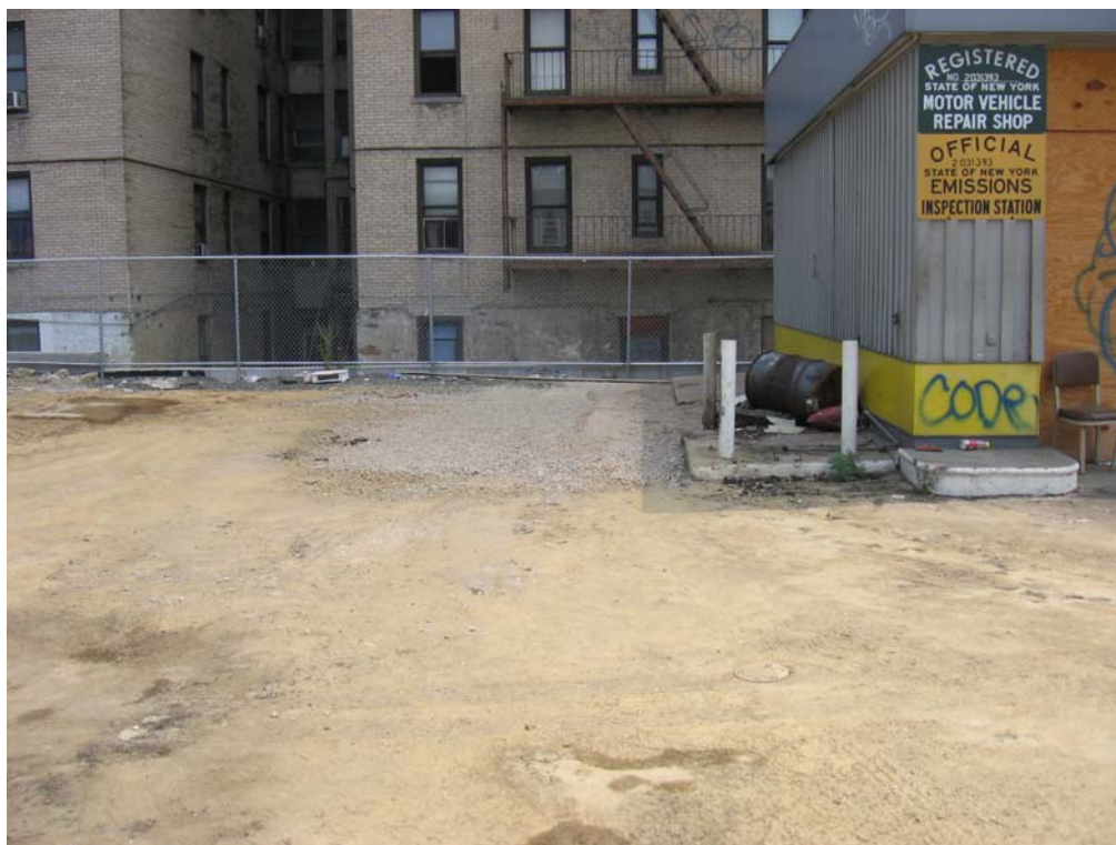
Backfilled Waste Oil Excavation
