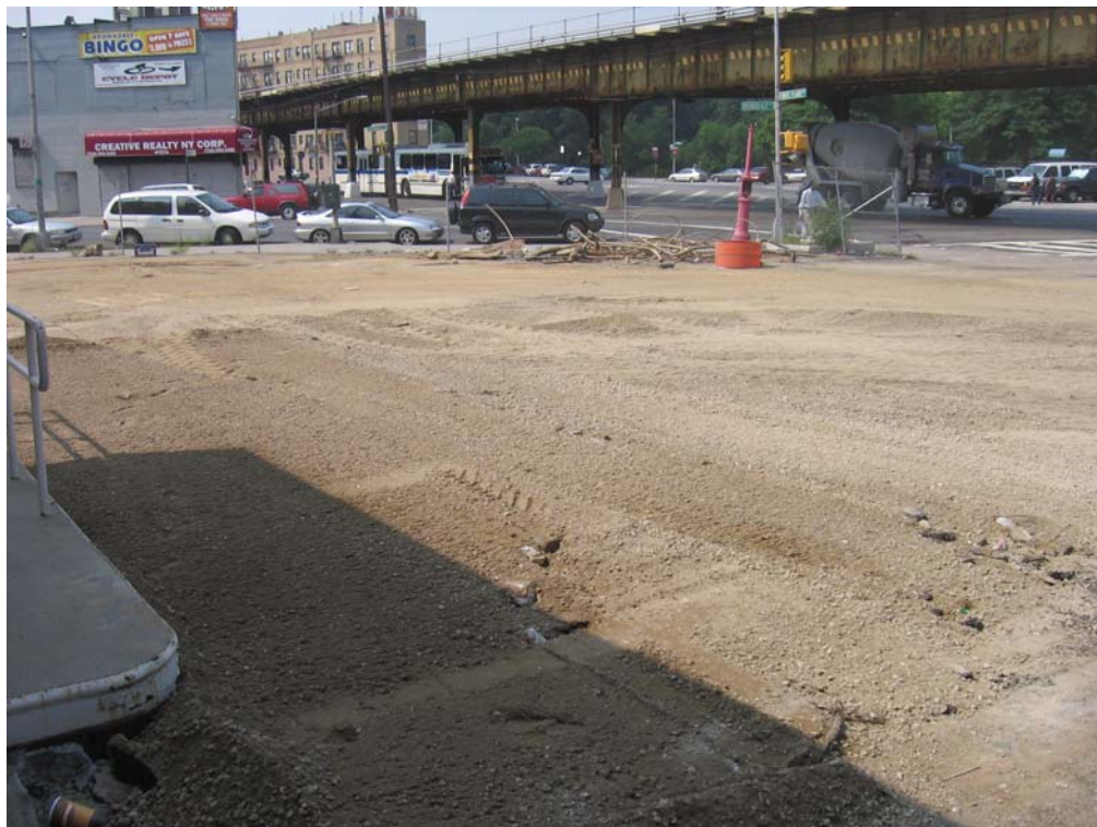
Backfilled Dispenser Excavation
