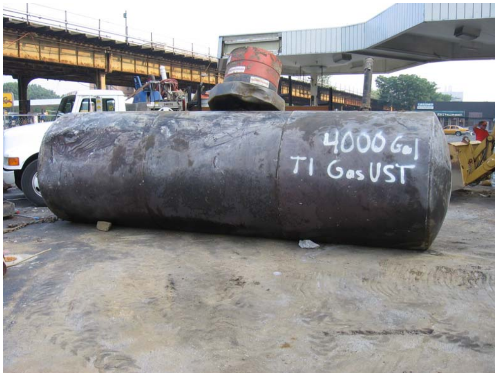
Tank1 – 4,000 gallon Gasoline UST
