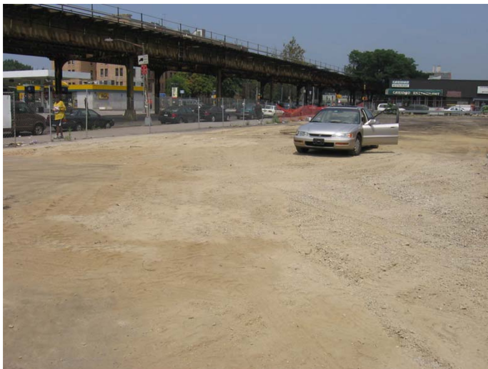
Backfilled Dispenser Excavation
