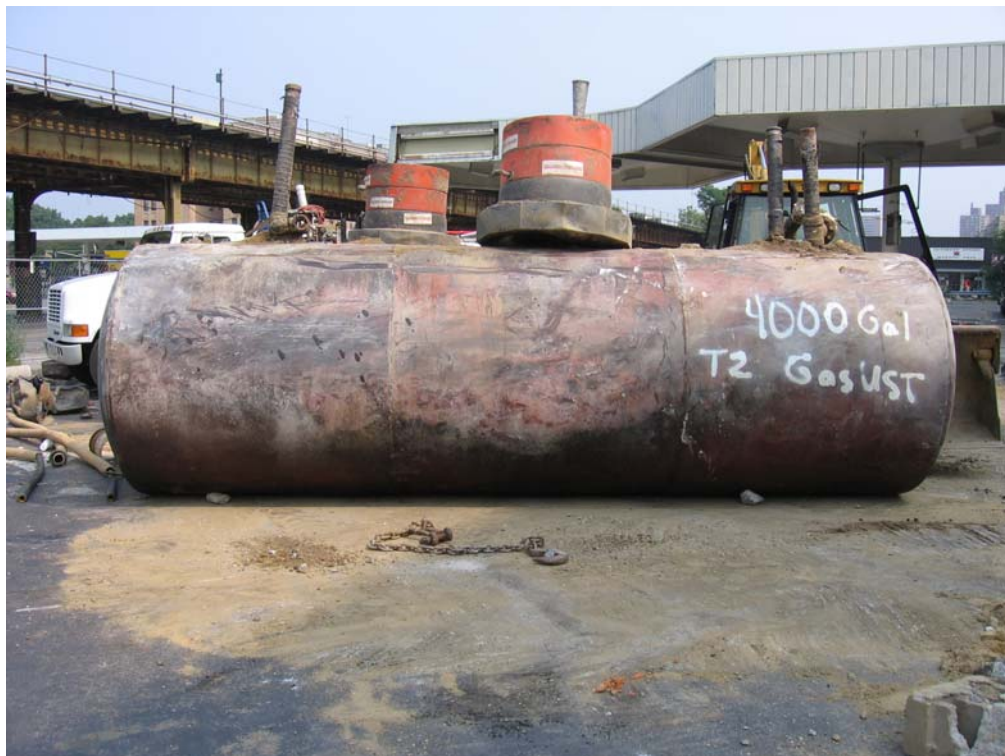
Tank2 – 4,000 gallon Gasoline UST
