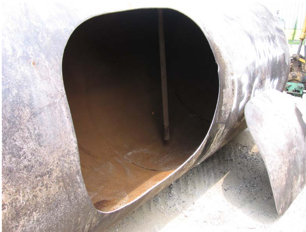
Tank3 – Interior of 4,000 gallon Gasoline UST
