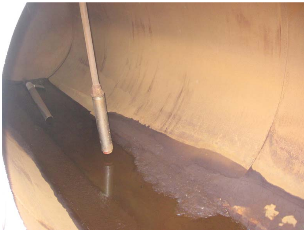
Tank1 – Interior of 4,000 gallon Gasoline UST
