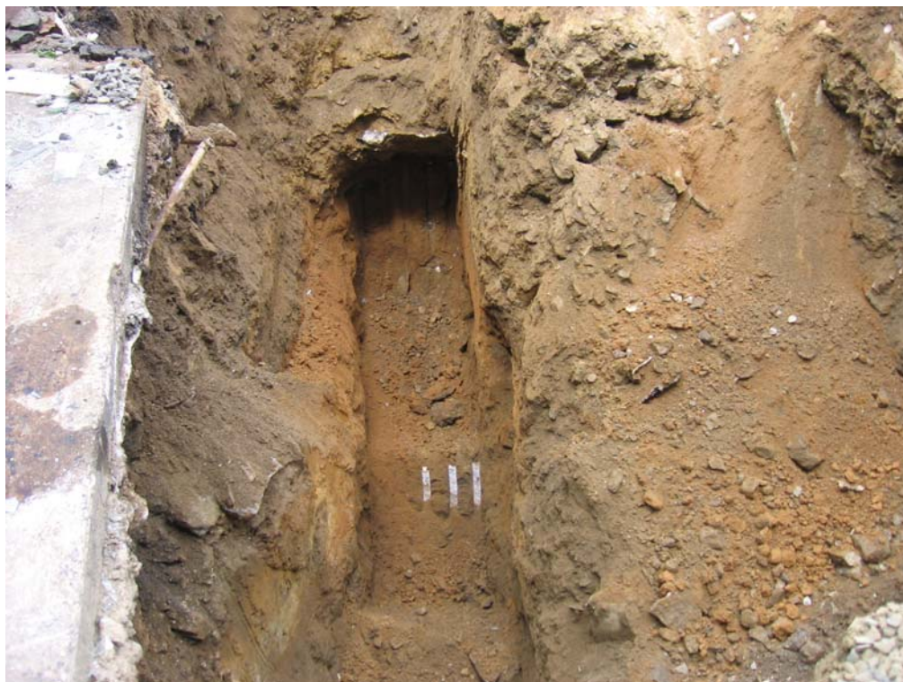
Bedrock Bottom of Waste Oil Excavation
