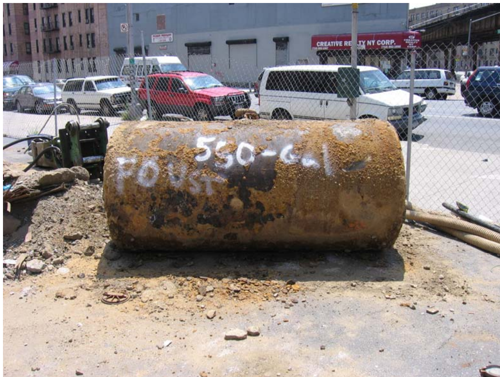
Tank4 – 550 gallon Fuel Oil UST
