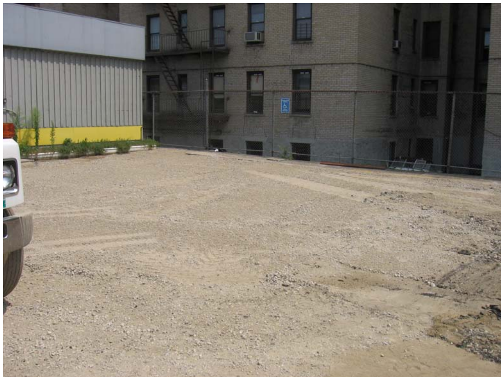
Backfilled UST Excavation
