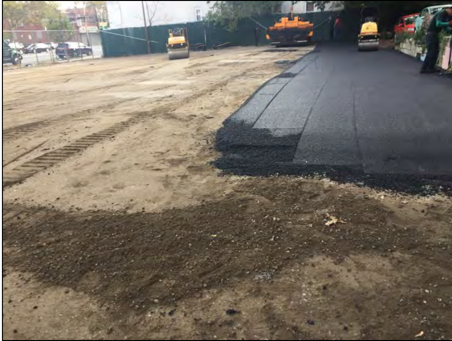
Photograph 15: Placement of 3.5 inch asphalt cover system.
