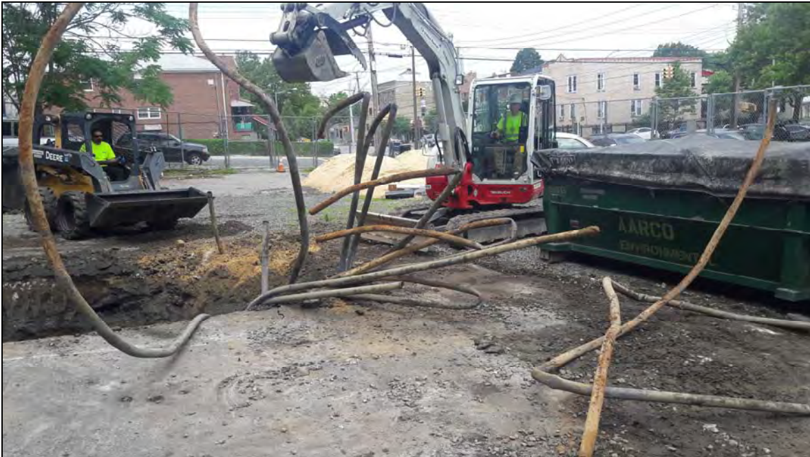
Photograph 9: Underground piping removal.
