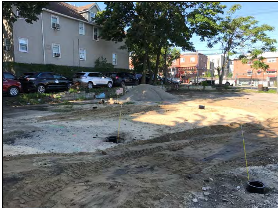
Photograph 13: Site preparation for capping with stockpiled sub-base material.
