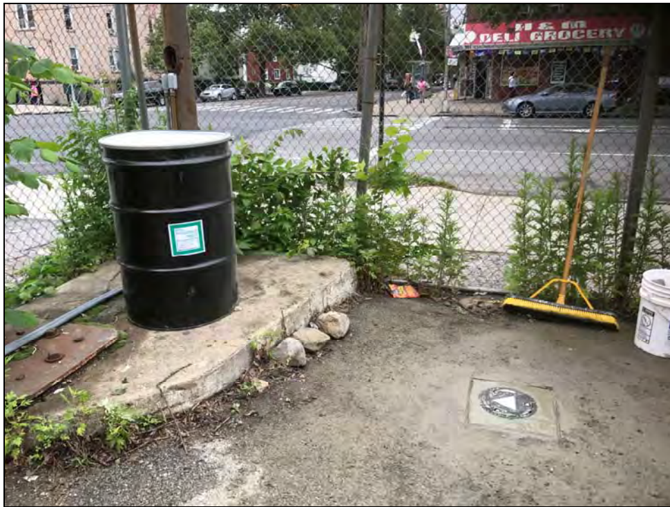
Photograph 3: Completed MW-13 with drummed derived waste (drill cuttings).
