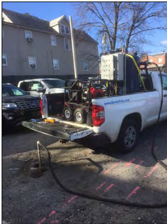
Photograph 1: Vacuum enhanced fluid recovery system for LNAPL recovery at MW-9.
