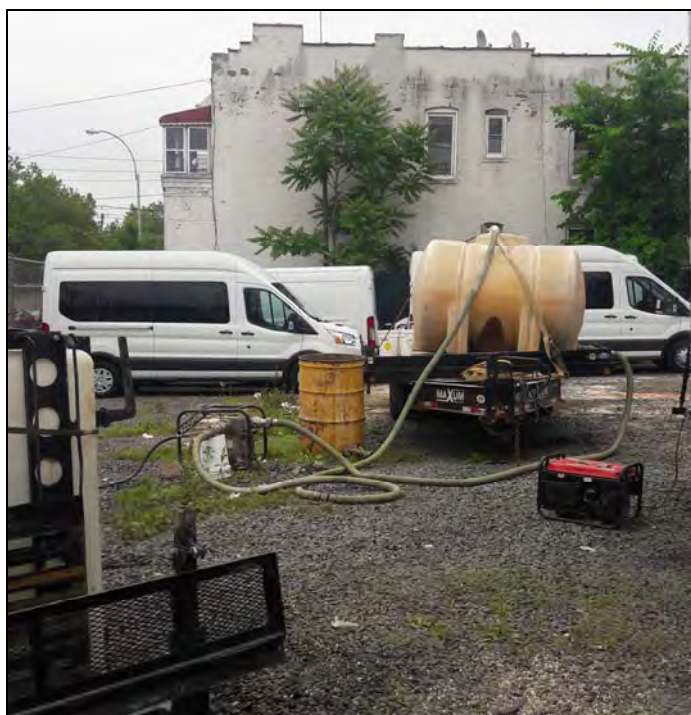
Photograph 6: Reagent delivery system set up.
