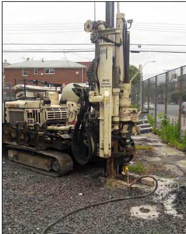
Photograph 5: Geoprobe rod advancement and reagent delivery at IP-9.
