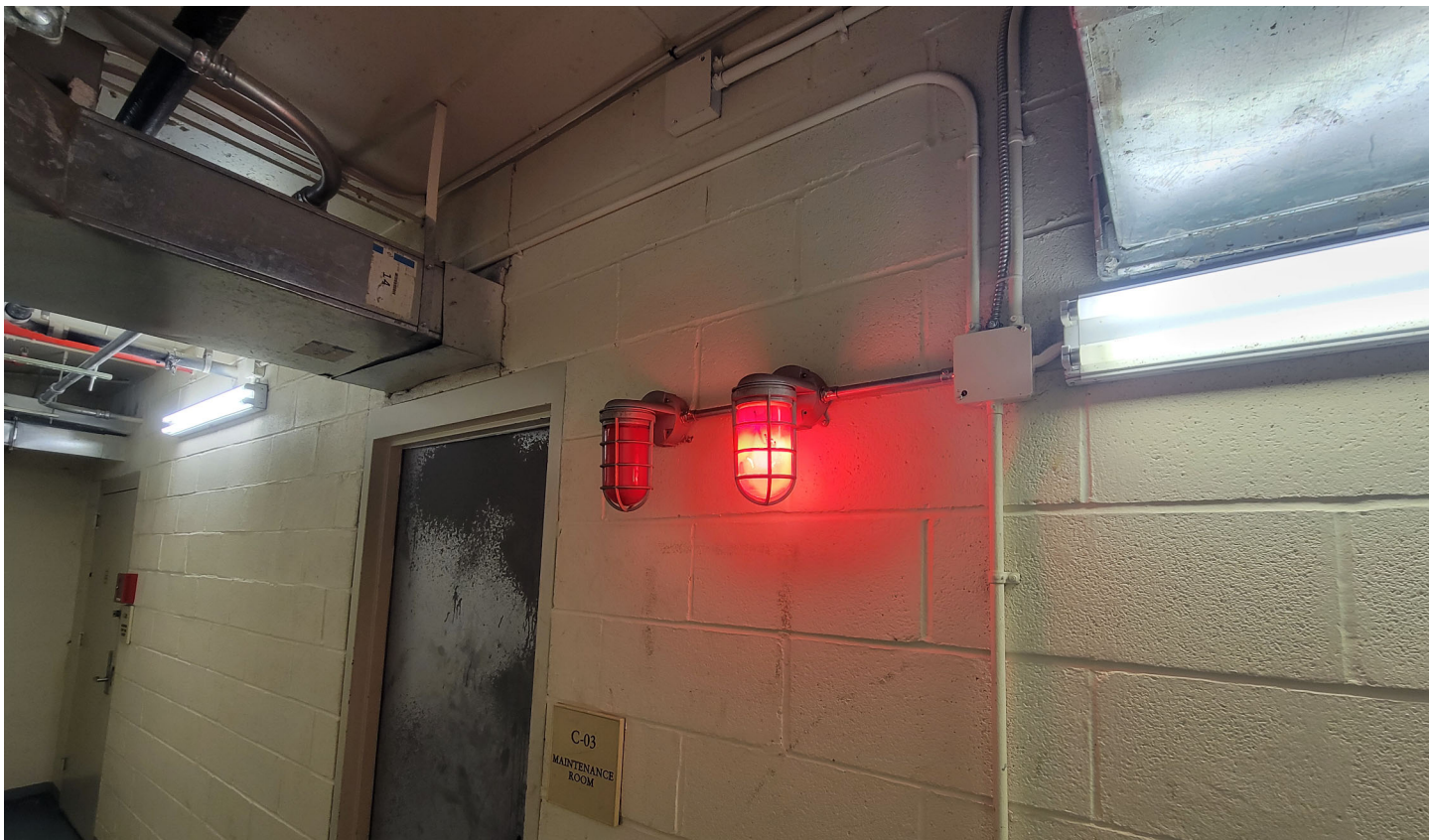
Testing of red alarm lights.
