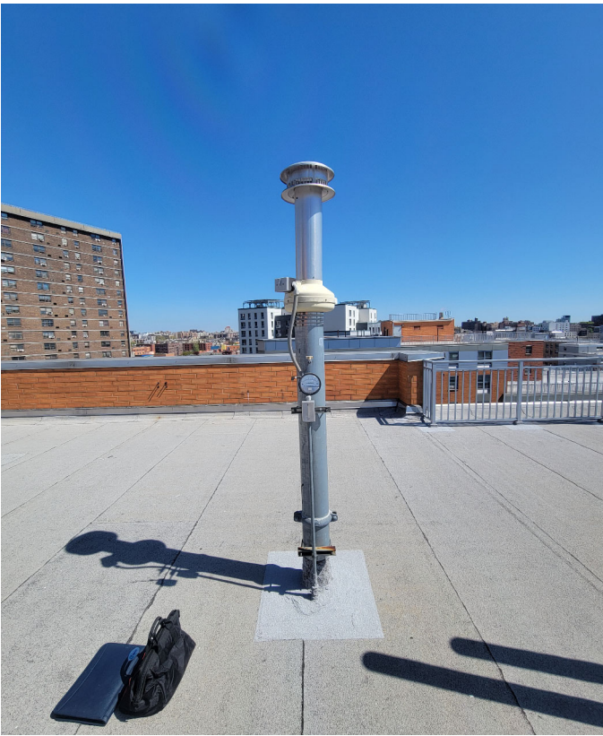
SSDS piping on 10th floor.
