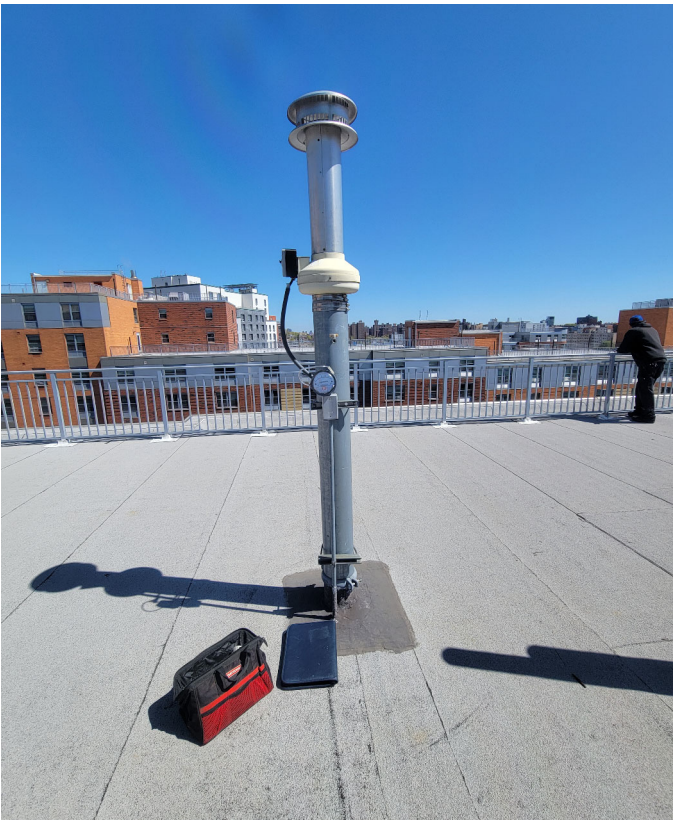
SSDS piping on the 8th floor.
