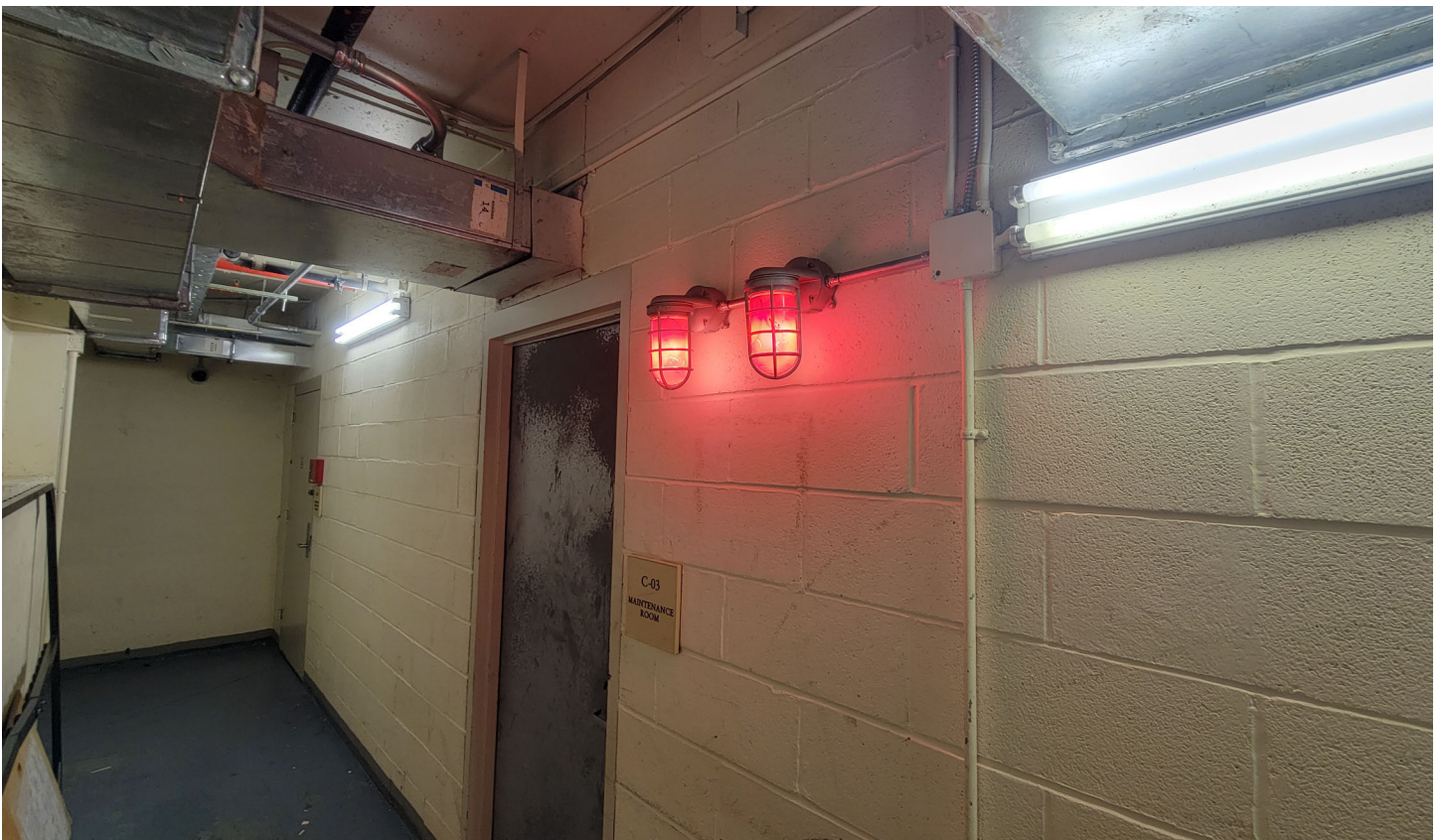
Testing of red alarm lights.
