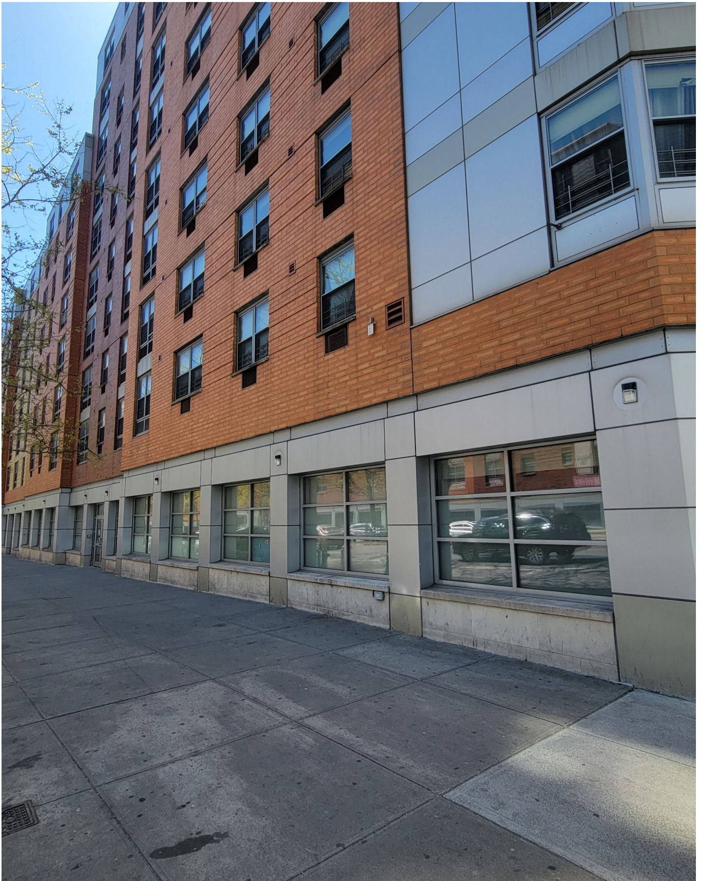
Site building along East 161st Street,
