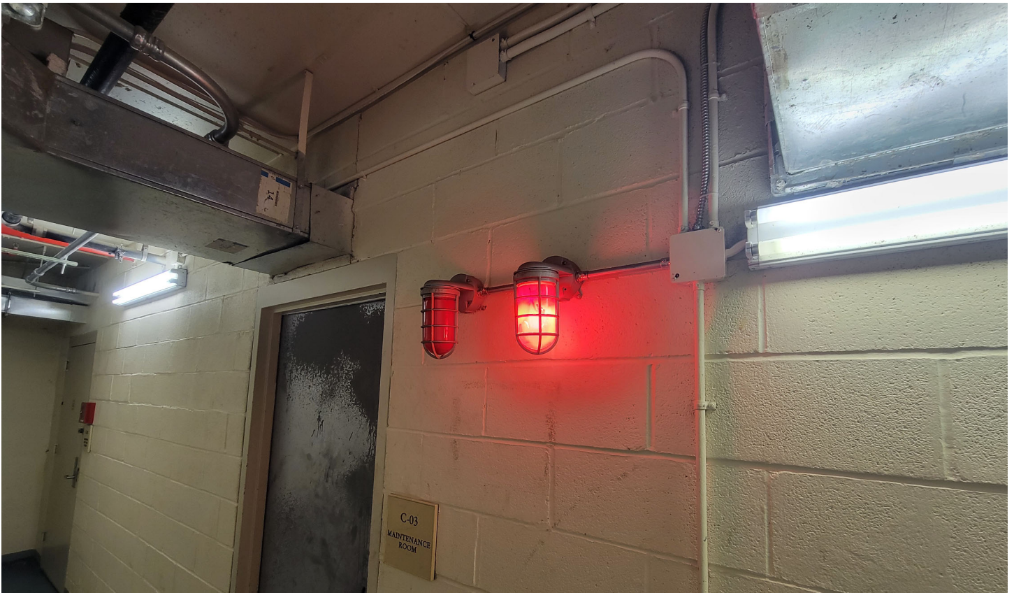
Testing of red alarm lights.
