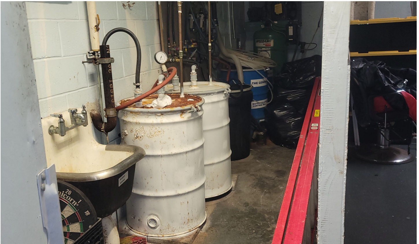
Groundwater pump and treat system
