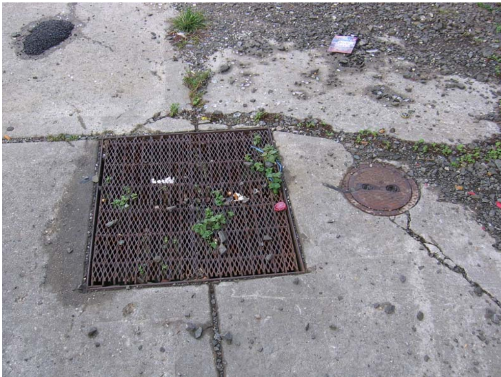
Photo 6: View of a sewer drain on the Site.
