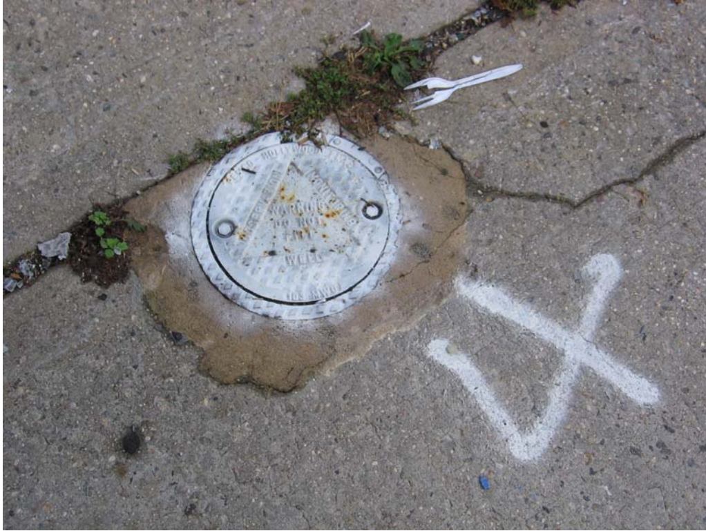
Photo 5: View of one of the four (4) water monitoring wells ATC observed on the Site.
