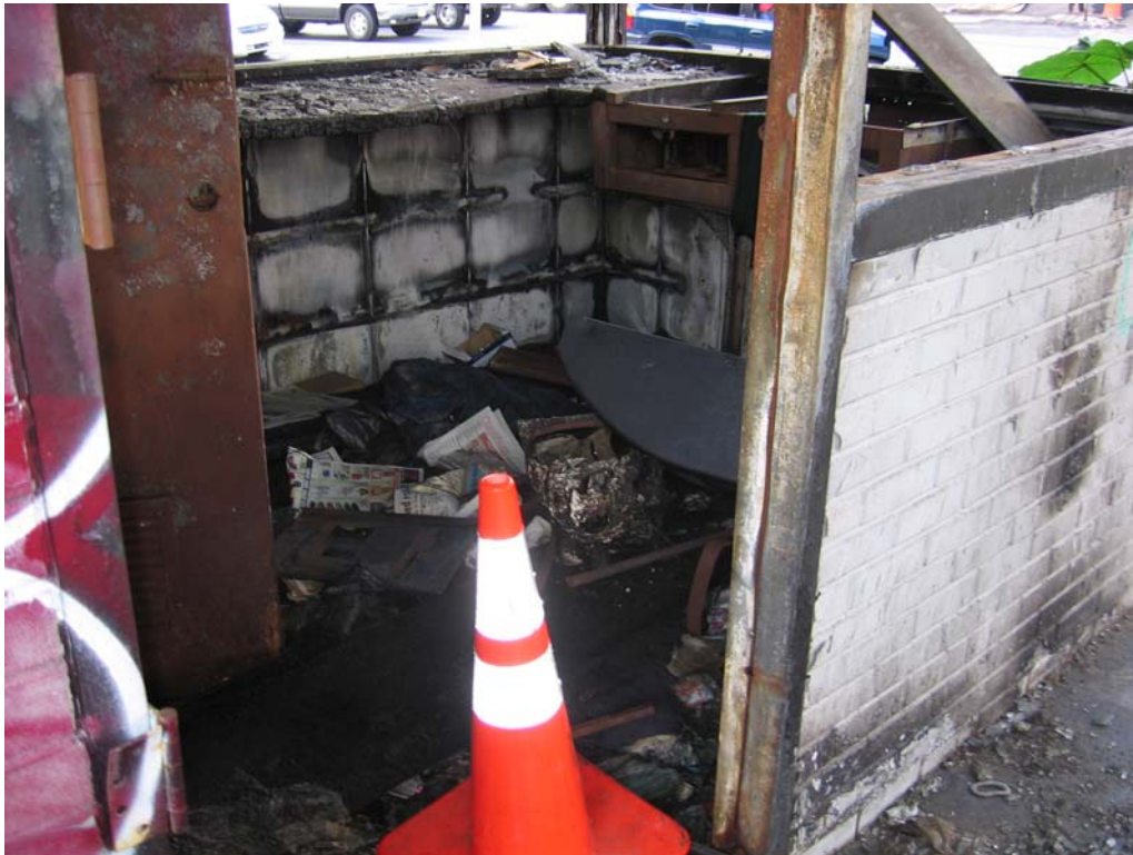
Photo 2: View of former attendant's booth on the Site.
