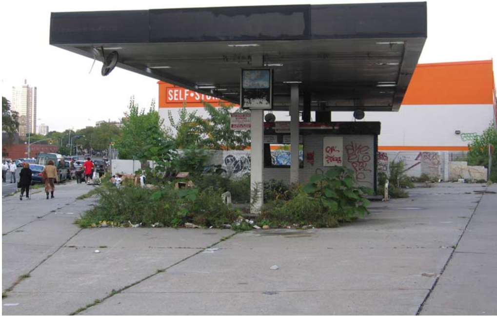
Photo 1: View of the Site from the south.
