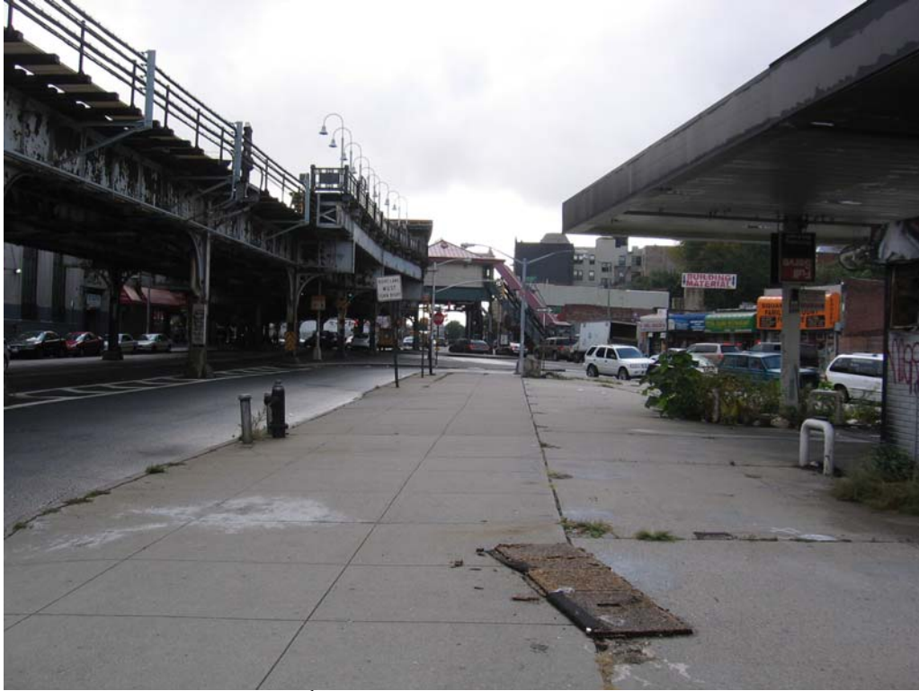
Photo 15: View of the 174 th Street subway station to the South down Boston Road.
