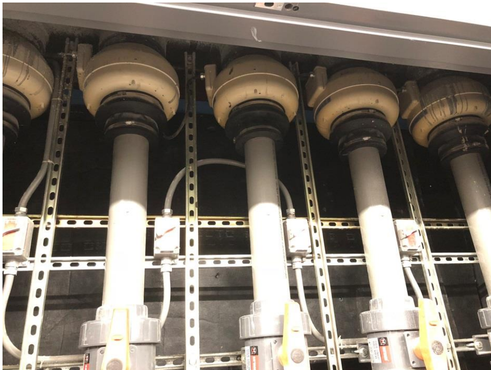
Photo 6 – View of SSDS blowers, located on the east mezzanine, facing east. Taken on 07/26/2018.
