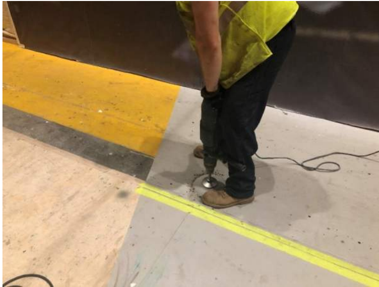
Photo 1: View of Eastern coring through the existing 10-inch-thick concrete slab, facing south.
