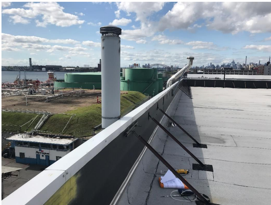
Photo 7: View of SSDS effluent exhaust stack on building roof, facing south. Taken on 09/13/2019.
