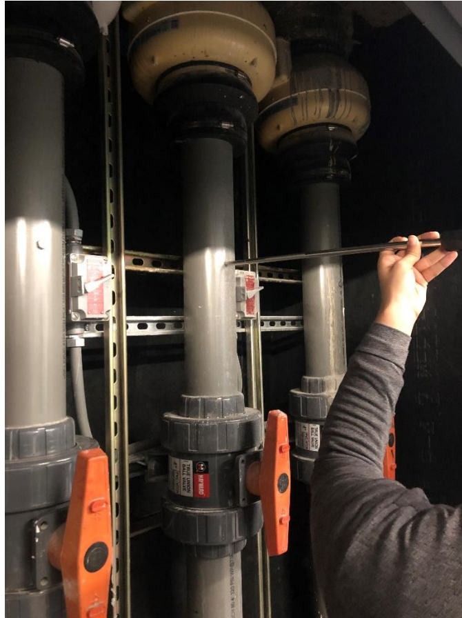
Photo 11: View of velocity reading collection from SSDS riser assembly, facing east. Taken on 12/30/2019.
