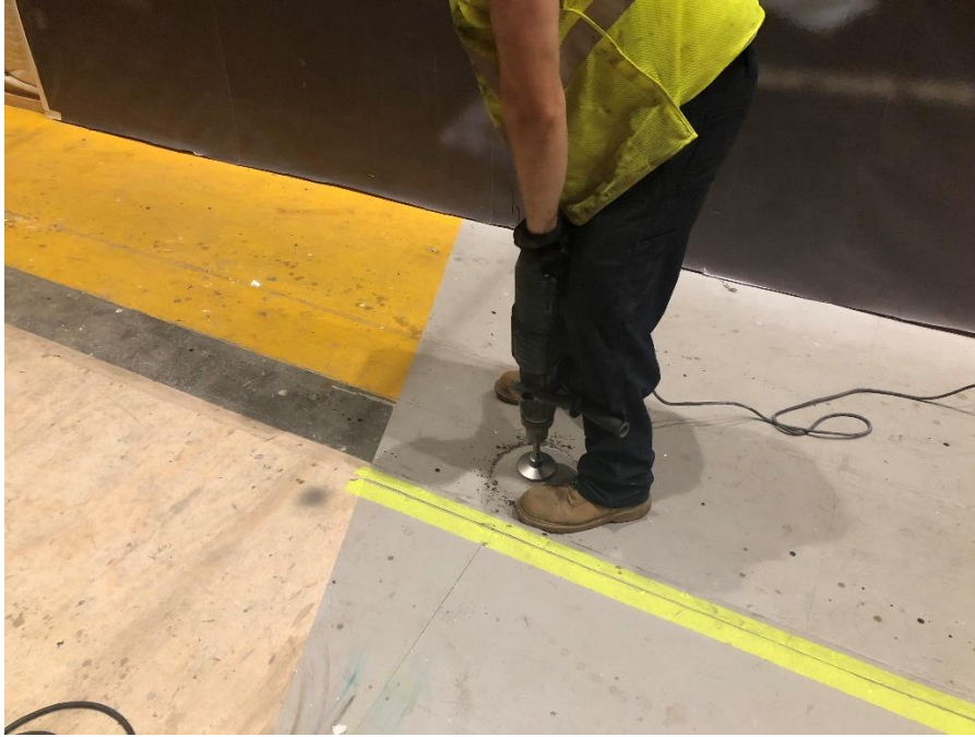
Photo 1: View of Eastern Environmental coring through concrete for installation of SVMF-08, facing east. Taken on 06/22/2019.
