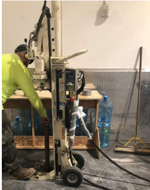
Photo 3: View of SVMF-04A installation using a direct push limited access rig, facing northeast.
