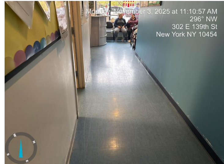
Photograph 10: Interior flooring in the Tres Puentes East Building, facing west.
