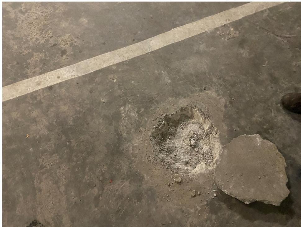
Photograph No. 4: Close-up of an area where concrete is chipped in parking garage.
