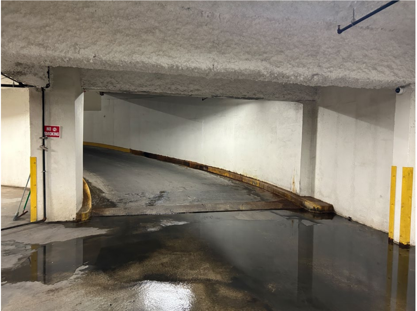
Photograph No. 1: View of the sub-grade parking garage ramp and sidewalls, facing northeast. Note: The ramp is part of the composite cover system in the Track 4 Remedial Area. Water is from a recent rain event.
