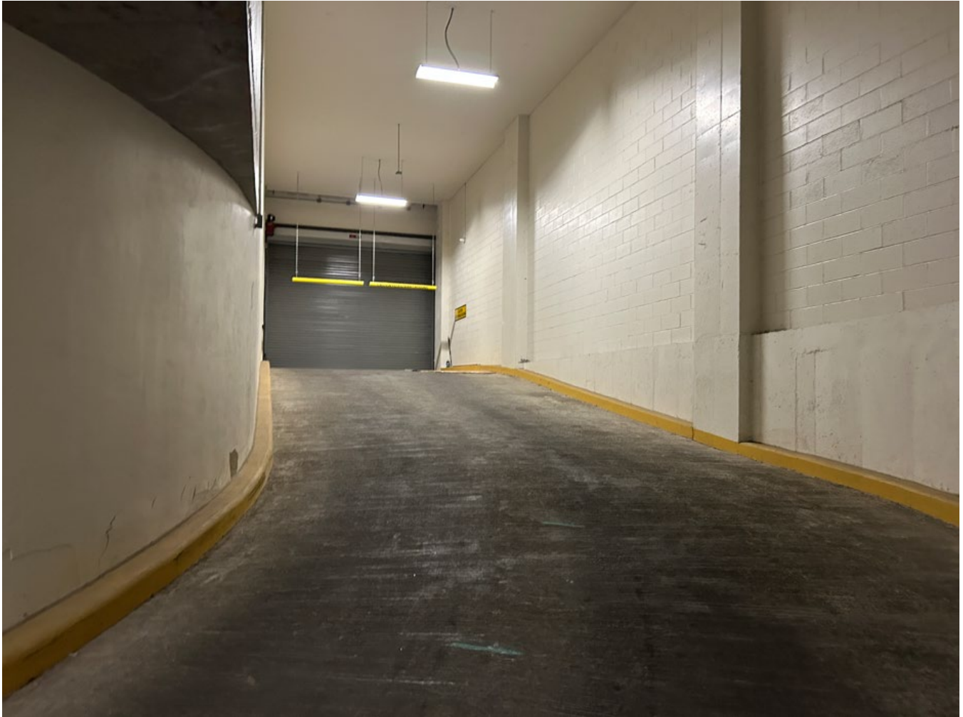
Photograph No. 2: View of the sub-grade parking garage ramp and sidewalls, facing northeast. Note: The ramp is part of the composite cover system in the Track 4 Remedial Area.
