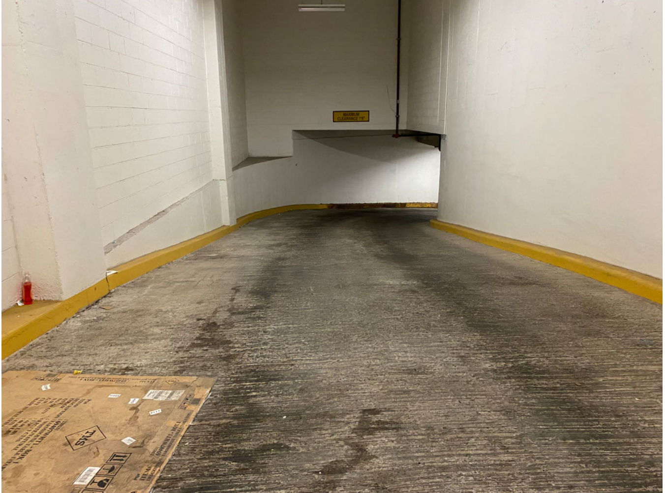
Photograph No. 2: View of the sub-grade parking garage ramp and sidewalls, facing southeast. Note: The ramp is part of the composite cover system in the Track 4 Remedial Area.
