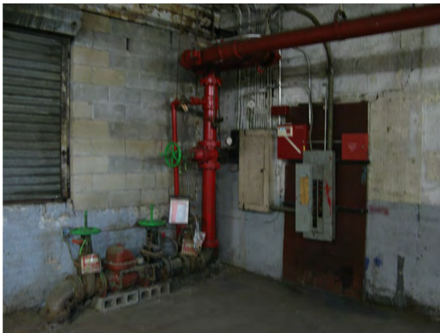
View showing fire sprinkler control valve assembly
