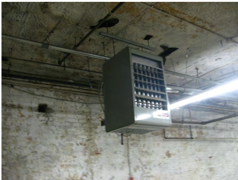
View of gas fired suspended heater
