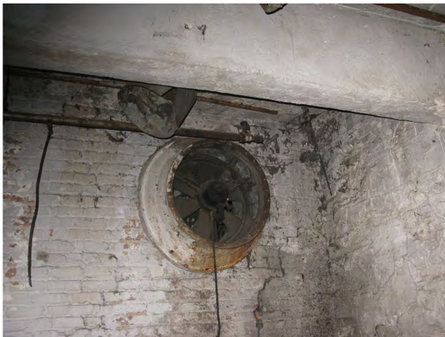
View showing wall mounted exhaust fan
