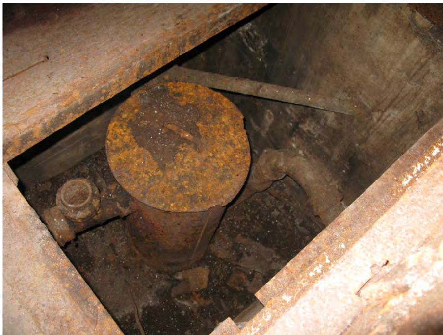
View showing sewer trap
