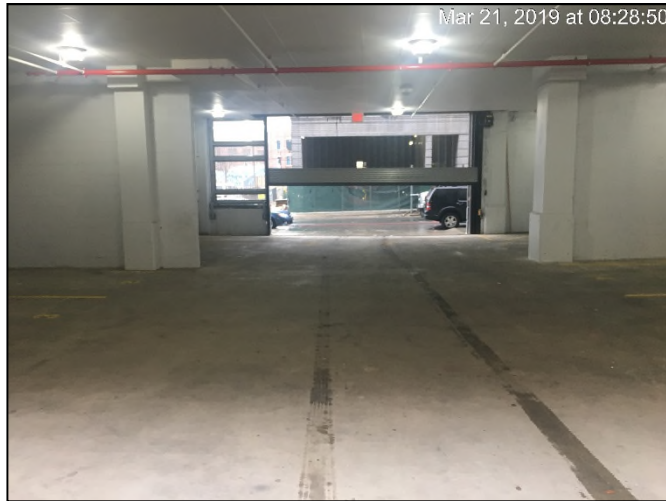
Photograph 1: Interior parking area on the northwestern portion of the Site.
