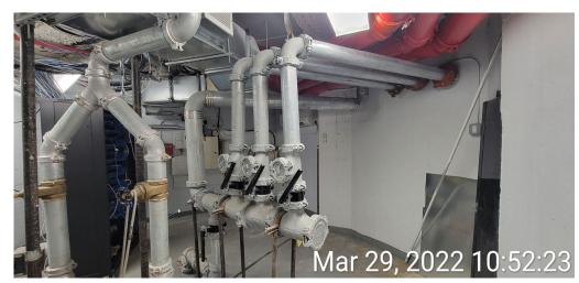
Photograph 14: Sub-slab depressurization system (SSDS) manifold in the cellar-level telecommunications room.
