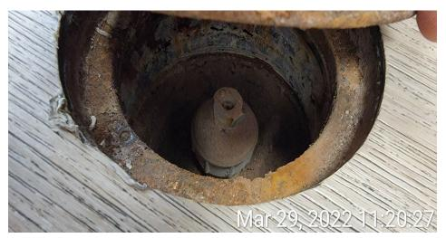
Photograph 13: Typical vapor monitoring point on the ground floor.
