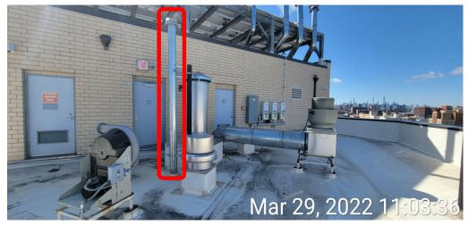
Photograph 15: SSDS exhaust stack with rain cap on the 12<sup>th</sup> floor roof.
