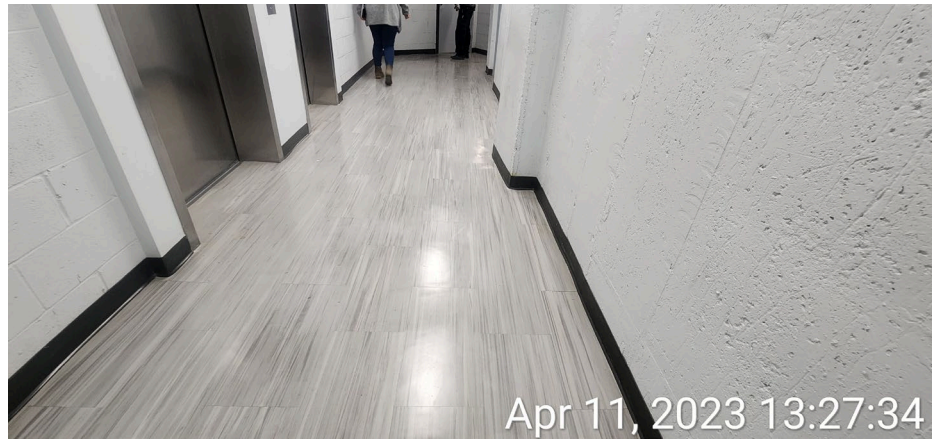
Photograph 10: Typical hallway finishing materials.
