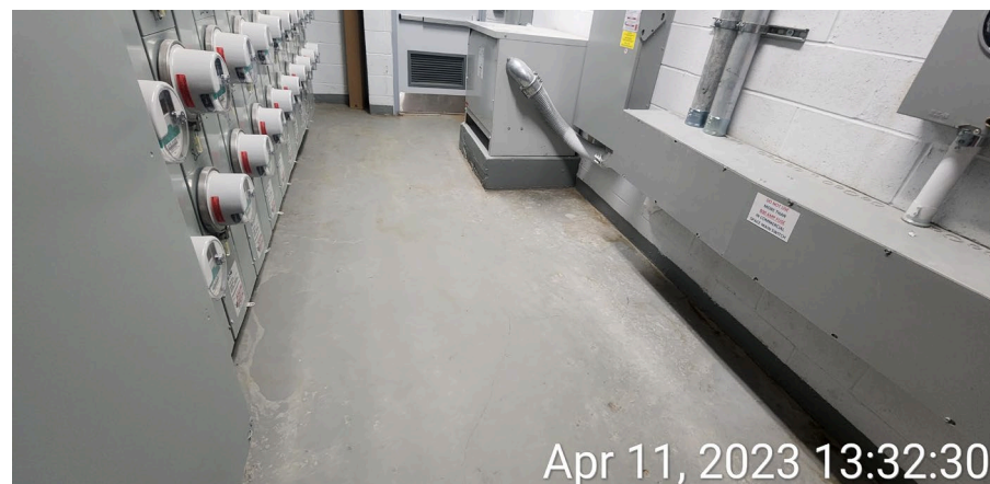
Photograph 8: Typical partial cellar slab in the cellar-level electric room.
