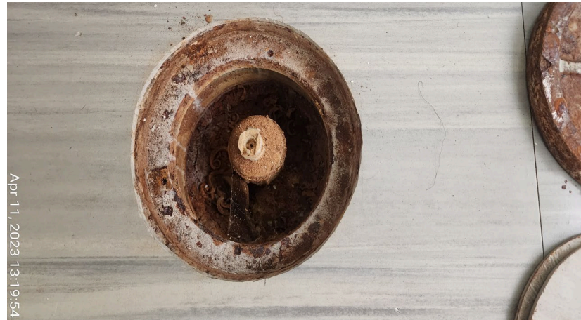
Photograph 13: Typical monitoring point on the ground floor.
