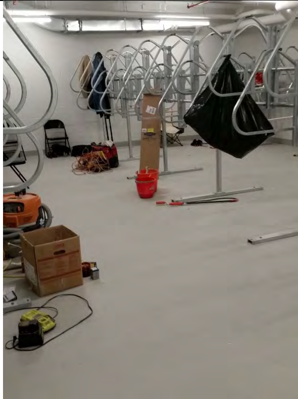
Photograph: 27 Interior Slab
