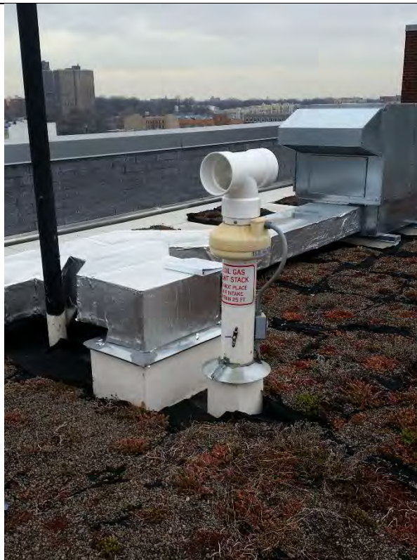
Photograph: 12 SP-03 access on roof exhaust stack
