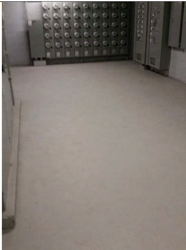
Photograph: 26 Interior Slab
