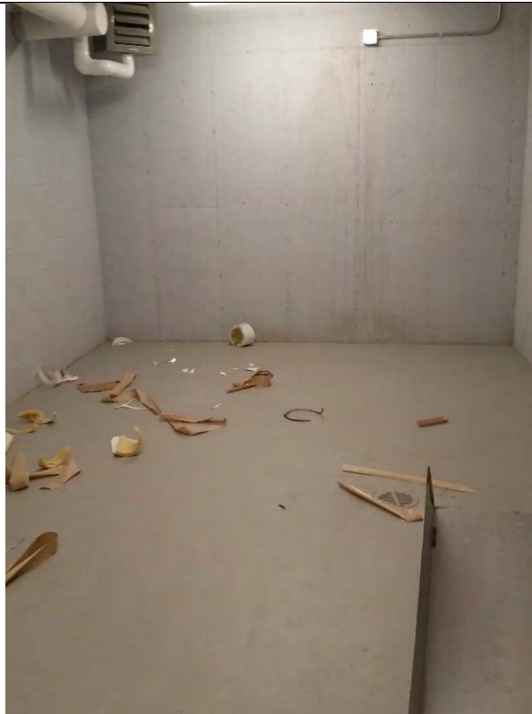
Photograph: 25 Interior Slab
