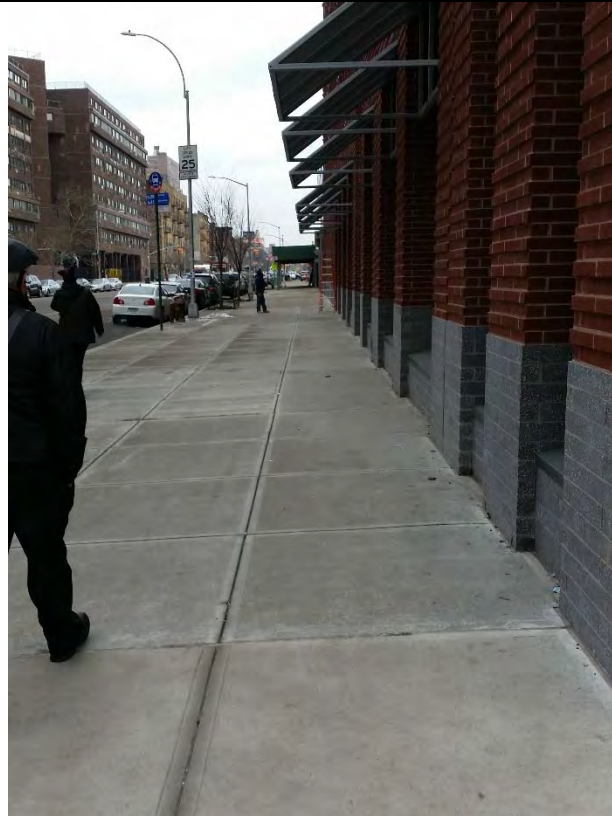
Photograph: 1 Building Exterior – East Side
