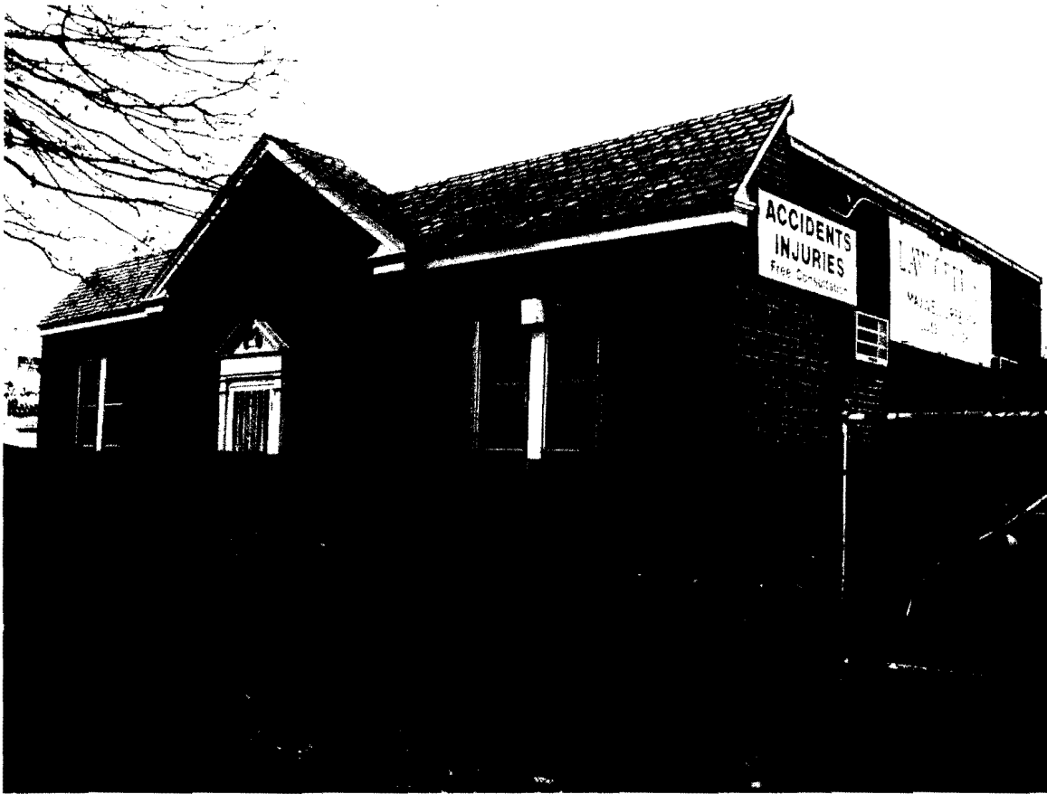
Adjacent Property to the East
