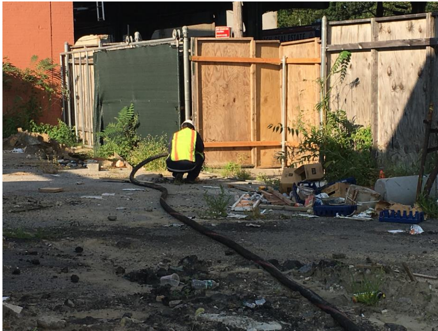
Photo 3: Brookside pumping out tank #1 with vacuum truck (facing southwest)
