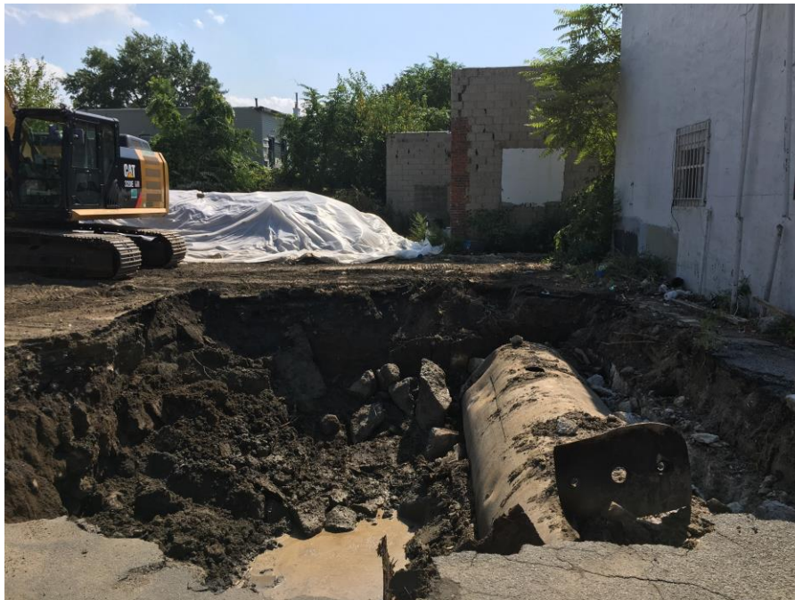
Photo 2: Exposure of 4,000-gallon UST and excavation area (facing south)
