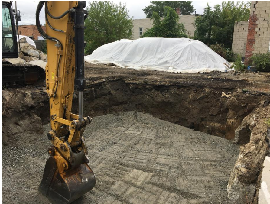
Photo 1: Backfill and compaction of RCA at AOC 2 (facing south)
