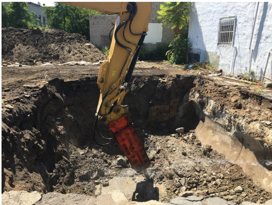
Photo 2: Hammering of concrete slab underneath former USTs (facing south)
