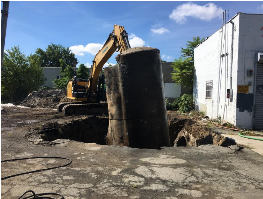
Photo 1: Removal of 4,000-gallon UST (facing south)
