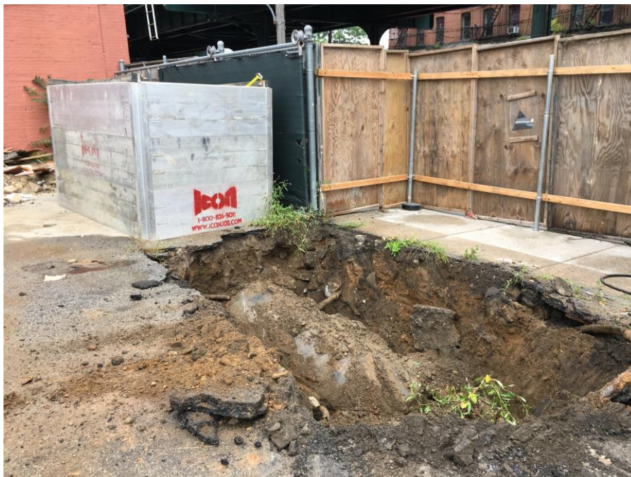
Photo 2: Exposure of 550-gallon UST at Tank Location 1 (facing northwest)
