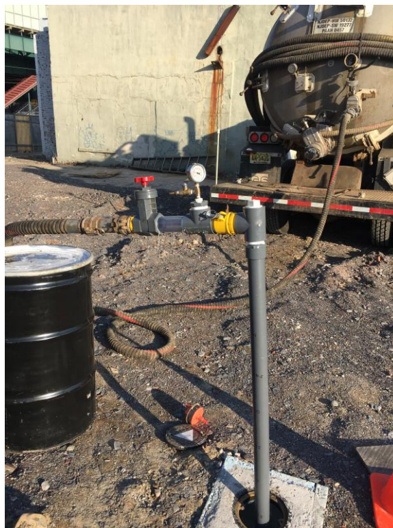
Photo 2: Wellhead assembly on stinger drop tube
