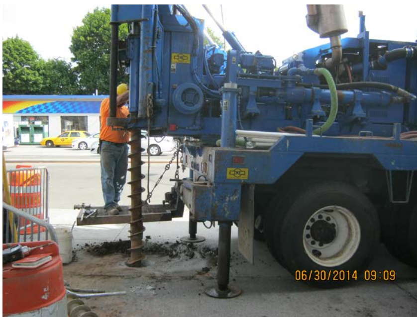
Photo 2: Location 1 during hollow-stem auger activities.
