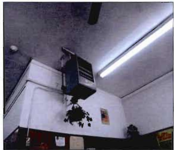
TYPICAL VIEW OF GAS FIRED CEILING HUNG HEATING UNIT
