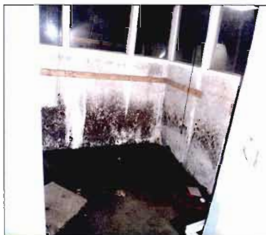
TYPICAL VIEW OF MOLD NOTED ON SITE
