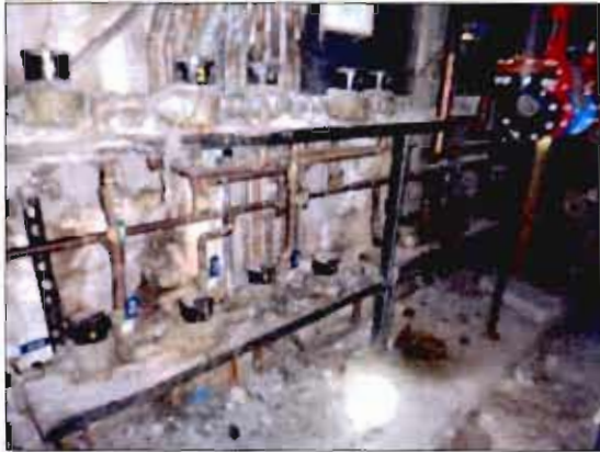
TYPICAL VIEW OF WATER MAIN AND METERS ON SITE
