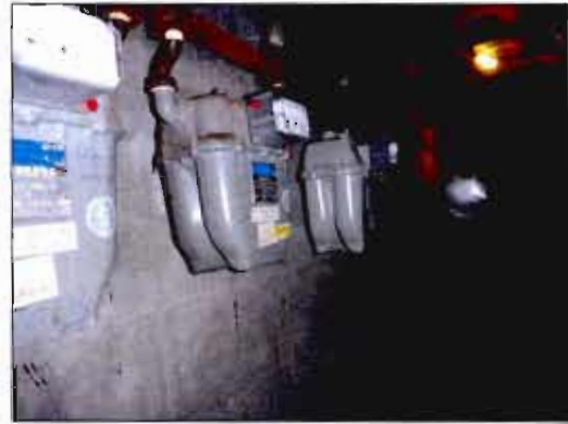
TYPICAL VIEW OF GAS MAIN WITH TENANT METERS FOUND ON SITE
