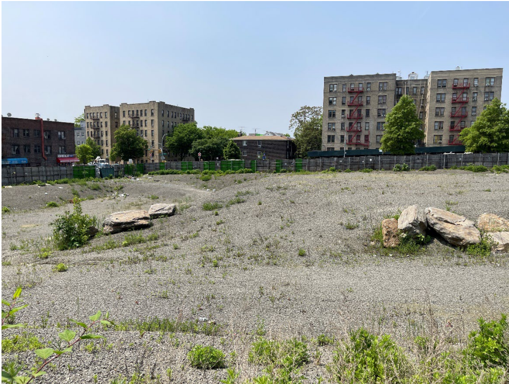
Photograph 1: Site Cover in place and comprised of soil cover consisting of a minimum of two feet of clean imported fill placed over a demarcation layer, with the upper six inches consisting of gravel.
