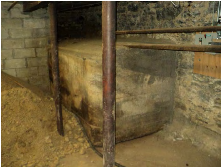
4. Concrete vaulted fuel-oil tank in the cellar of the ministry building
