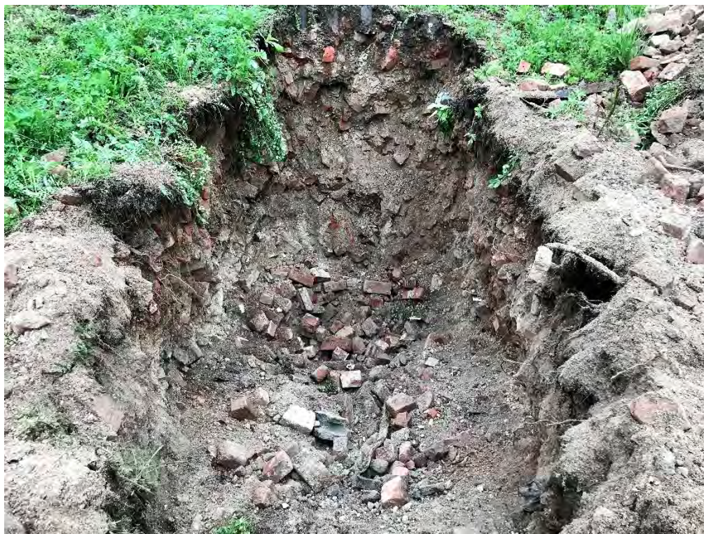
Photo 10: TP-10 in WC-4 – Fill material consisting of brick, concrete, and metal debris.
