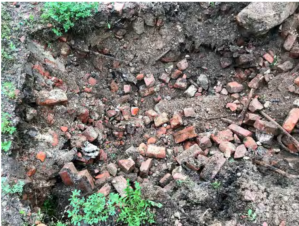
Photo 6: TP-6 in WC-4 – Fill material consisting of brick, concrete, metal debris, and trace coal/slag.
