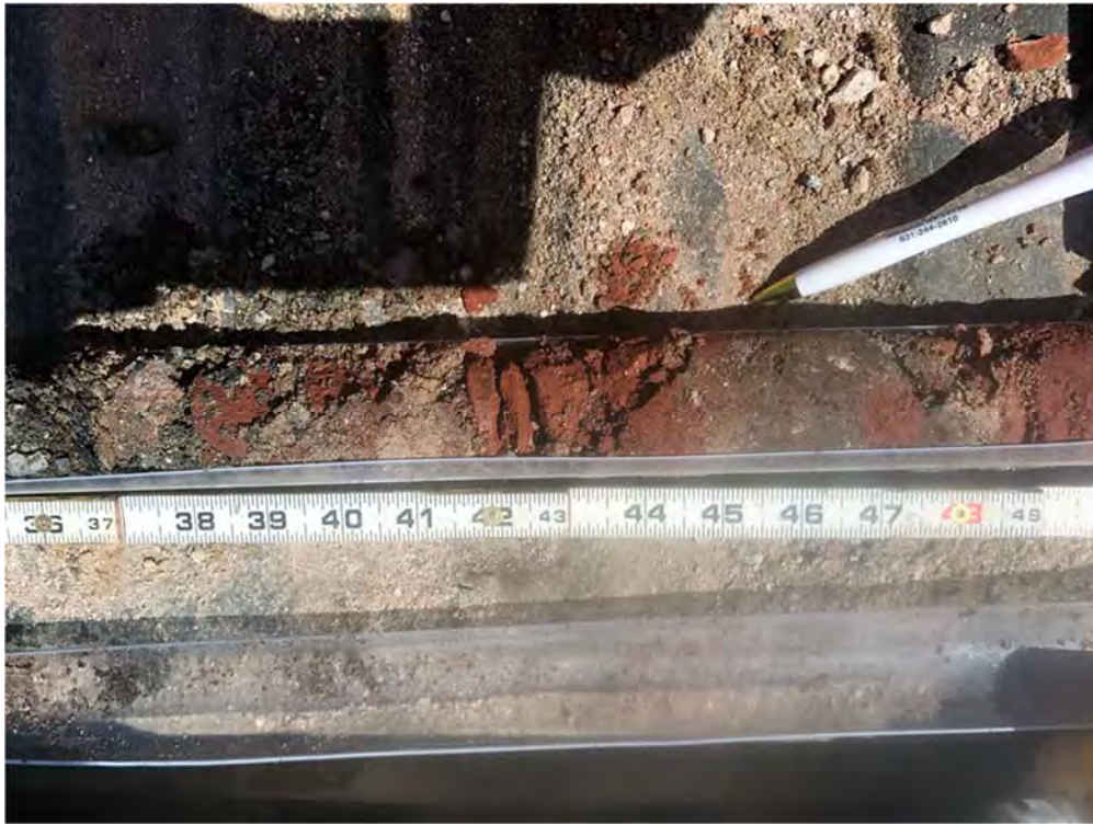
Photo 13: SB-2 (0-5') in WC-1 – Fill containing brick, concrete, and trace coal/slag.
