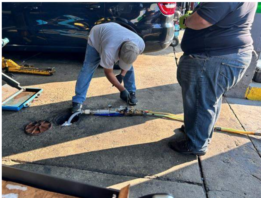
Photo 2: Endeavour filling the UST with Tripolymer® 105 Tank Media Resin (facing north).
