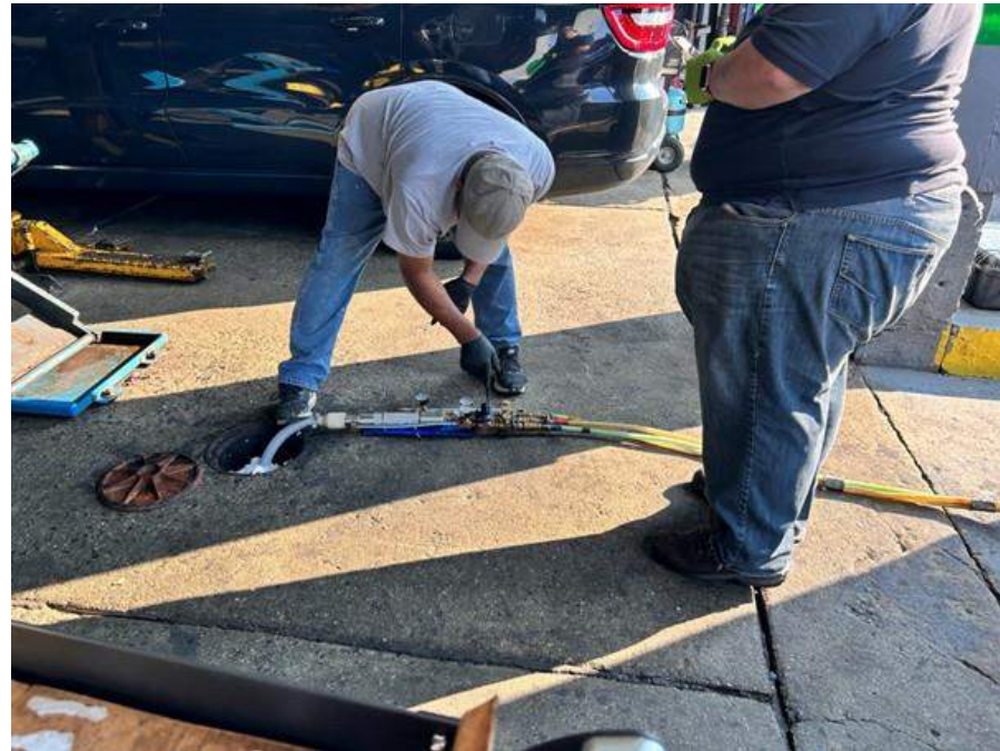
Photo 2: Endeavour filling the UST with Tripolymer® 105 Tank Media Resin (facing north).
