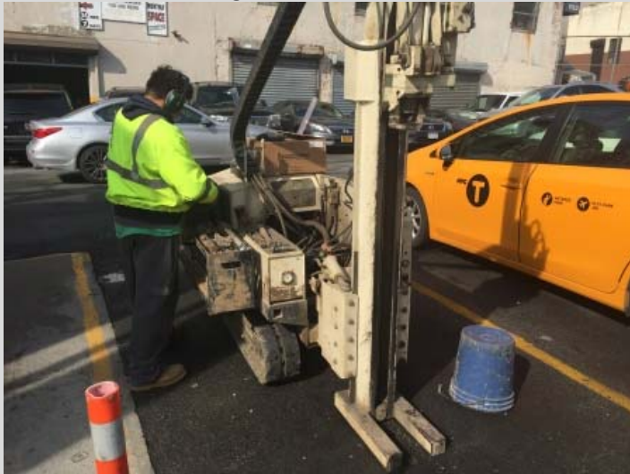
PHOTO 9: B-16 Boring Location
