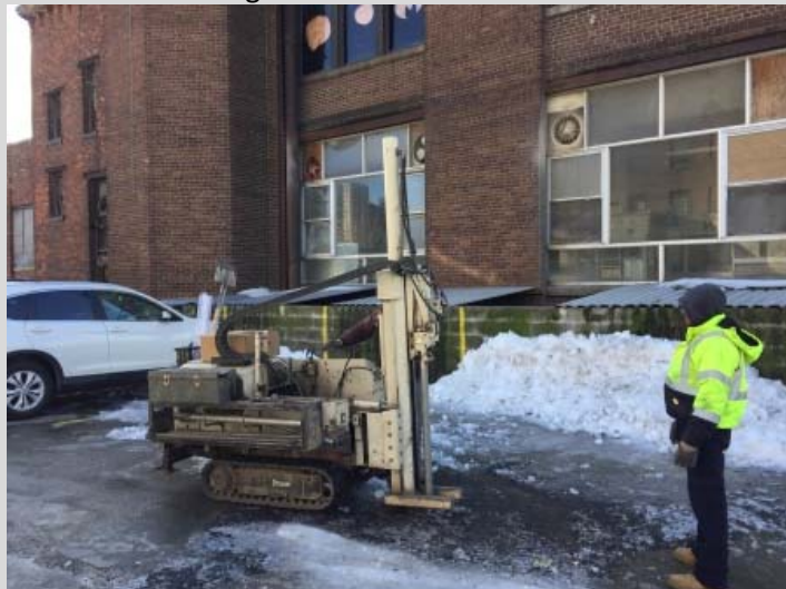
PHOTO 13: Drilling Location at B-23
