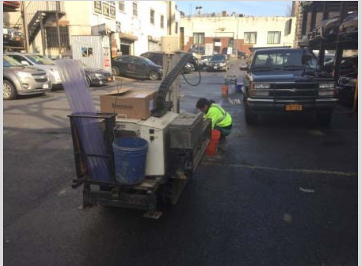
PHOTO 4: B-13 Boring Location
