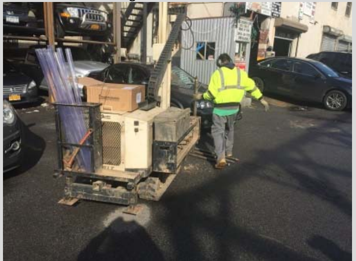
PHOTO 6: B-14 Boring Location
