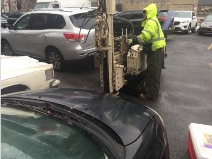
PHOTO 1: Drilling Location at B7
