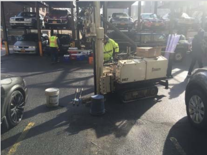
PHOTO 5: B-14 Boring Location
