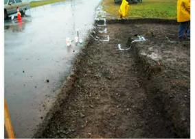
Picture 1: Sidewalk excavation and bollard layout
