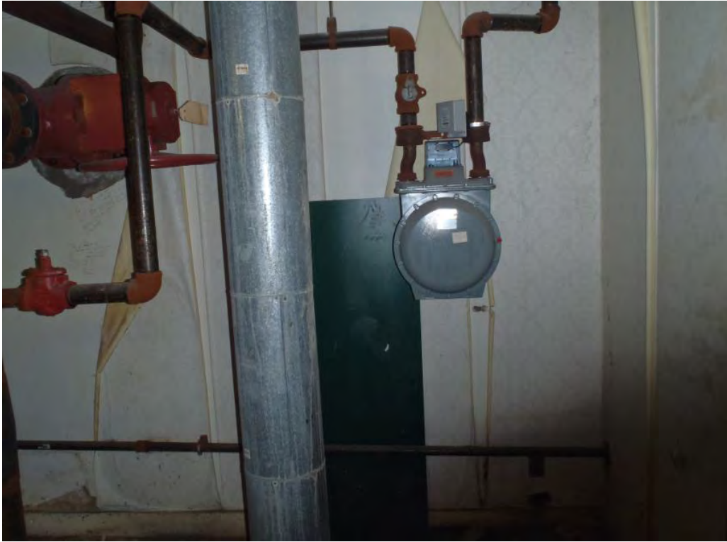
Photo 13: View of the natural gas meter observed in the basement of the building.
