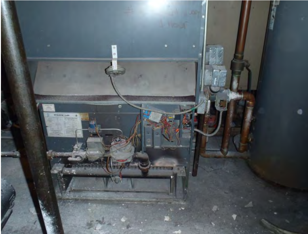
Photo 11: View of the natural gas fired furnace observed in the basement of the building.
