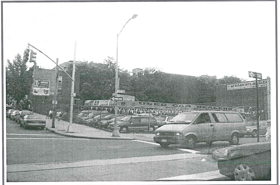
Photograph Number 1: View of the Property from the intersection of Park Avenue and E 168 th Street.
