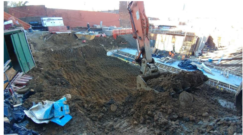
Photograph 12. Excavation continues for the remaining cellar step-footings.
