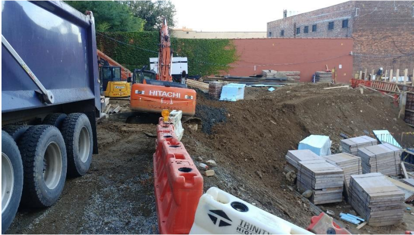
Photograph 9. Site excavation/direct-loading of trucks with soil for off-site disposal.
