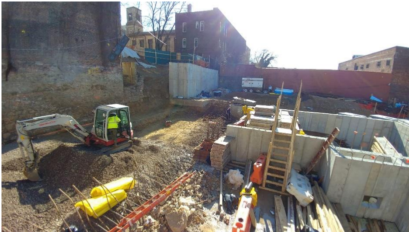
Photograph 17. Moncon removes the 3/4" stone blend from behind the western wall in Grids A1 and A2, per the corrective action work plan (CAWP).
