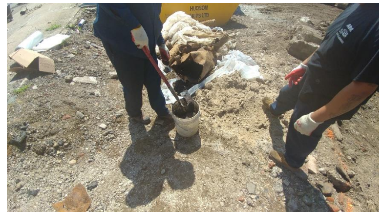
Photograph 4. ABC Fuel Oil Cleaners were mobilized to clean and dispose of the tank and piping, and drum of contaminated soil from inside the tank.
