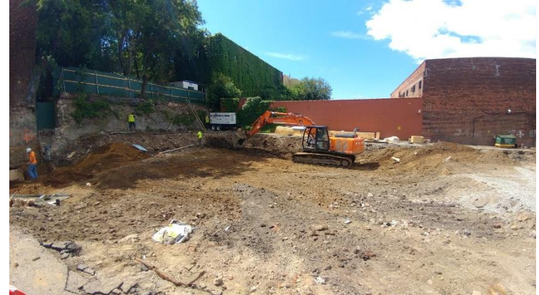
Photograph 2. Excavation activities begin on the site (viewing grids B1, B2, C1, and C2).
