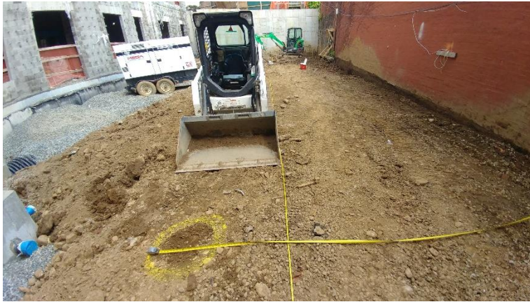
Photograph 21. AKRF collects post-excavation endpoint samples from Grid B2 and measures endpoint sampling locations.
