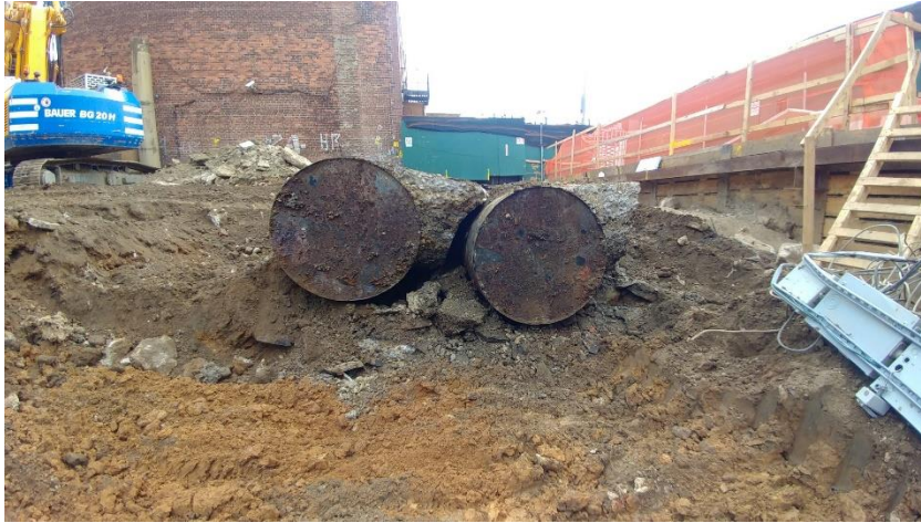
Photograph 5. Two 550-gallon USTs were discovered in Grids A1 and A2 during excavation and SOE work.
