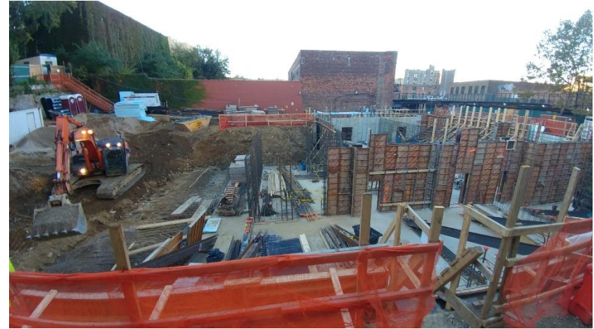
Photograph 10. Clean imported stone is spread for the step-footings in Grid B1. Concrete forms are installed for future concrete wall pours.
