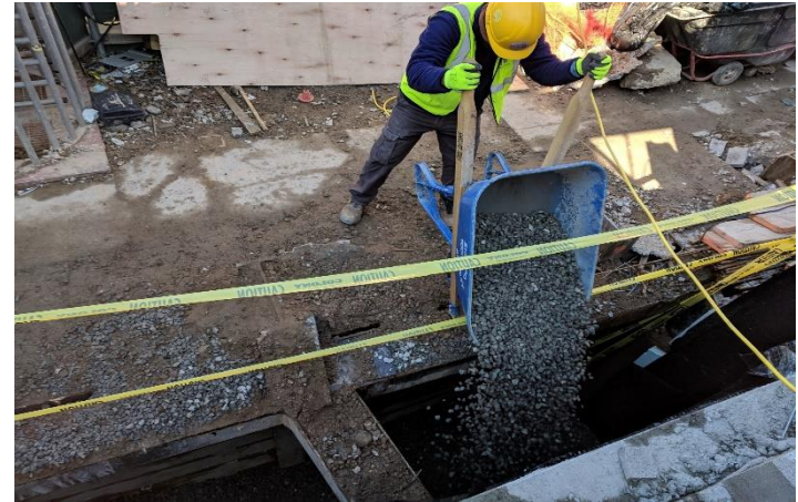
Photograph 18. The 3/4" stone blend is replaced with virgin stone behind the western wall in Grids A1 and A2.
