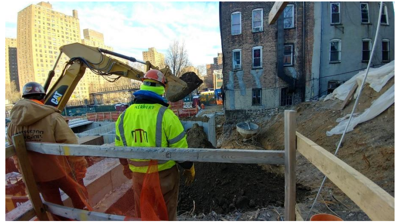
Photograph 16. The temporarily staged off-site soil is placed behind the new retaining wall (off-site) behind the new soil retaining wall.
