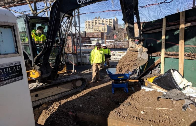
Photograph 17. Moncon removes the 3/4" stone blend from behind the western wall in Grids A1 and A2, per the corrective action work plan (CAWP).
