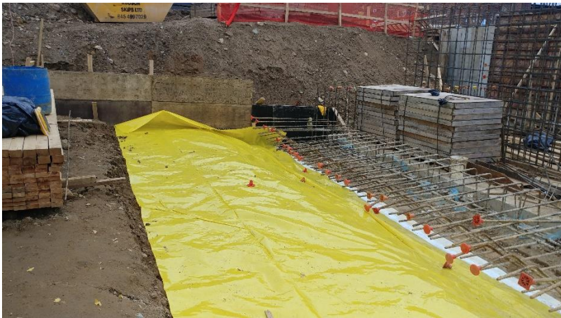
Photograph 11. Mega installed Stego Wrap vapor barrier for the Grid B1 step footing and connected it to the Grace Preprufe waterproofing membrane in the Grid A1/A2/B1.
