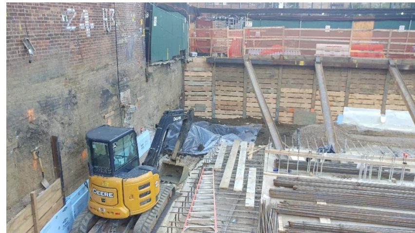
Photograph 8. During foundation excavation and rebar installation activities, contaminated soil discovered in Grid A2 was excavated and covered until it could be properly disposed of.
