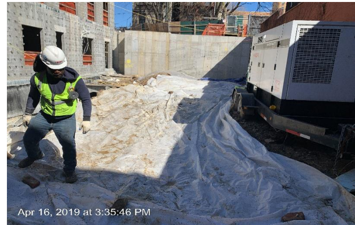
Photograph 20. Plastic sheeting was placed over exposed soil in the rear yard when subsurface disturbance was not occurring.
