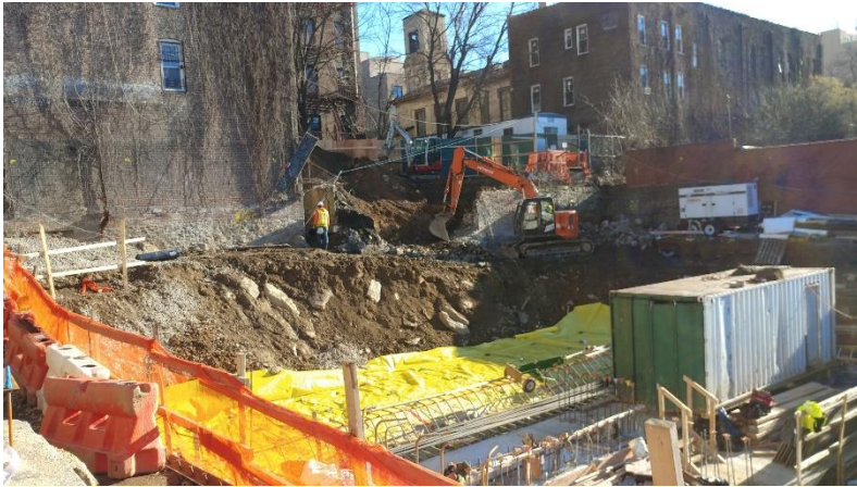
Photograph 13. Moncon demolishing the retaining wall on the eastern property boundary.
