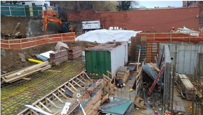
Photograph 15. Moncon covers off-site soil stockpile with plastic sheeting in Grids C2 and B2.
