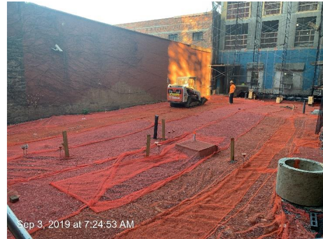
Photograph 22. Mega installs a demarcation barrier consisting of orange snow fence within Grids B2 and C2.
