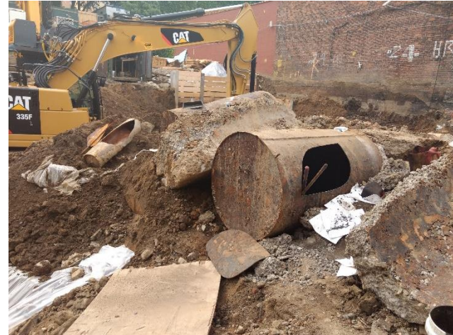
Photograph 6. Brookside Environmental pumped out, cleaned, and removed the USTs from the site.
