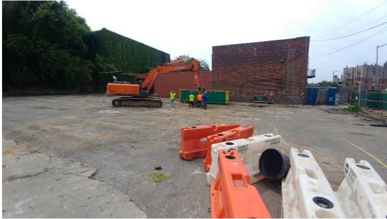
Photograph 1. The site is cleared of debris prior to excavation activities.
