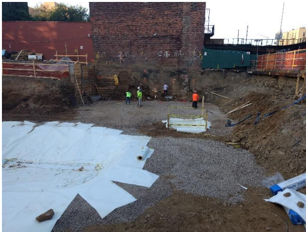
Photograph 7. Following initial end point sampling, clean stone was imported and Grace Preprufe 300R was installed in Grids A1, A2, and B1.
