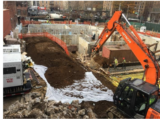
Photograph 14. Due to space constraints, Moncon temporarily stages off-site soil that fell down during demolition of the retaining wall.
