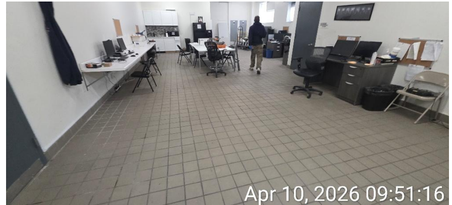
Photograph 4: The ground floor offices in the Track 4 portion of the Site, view facing northwest.
