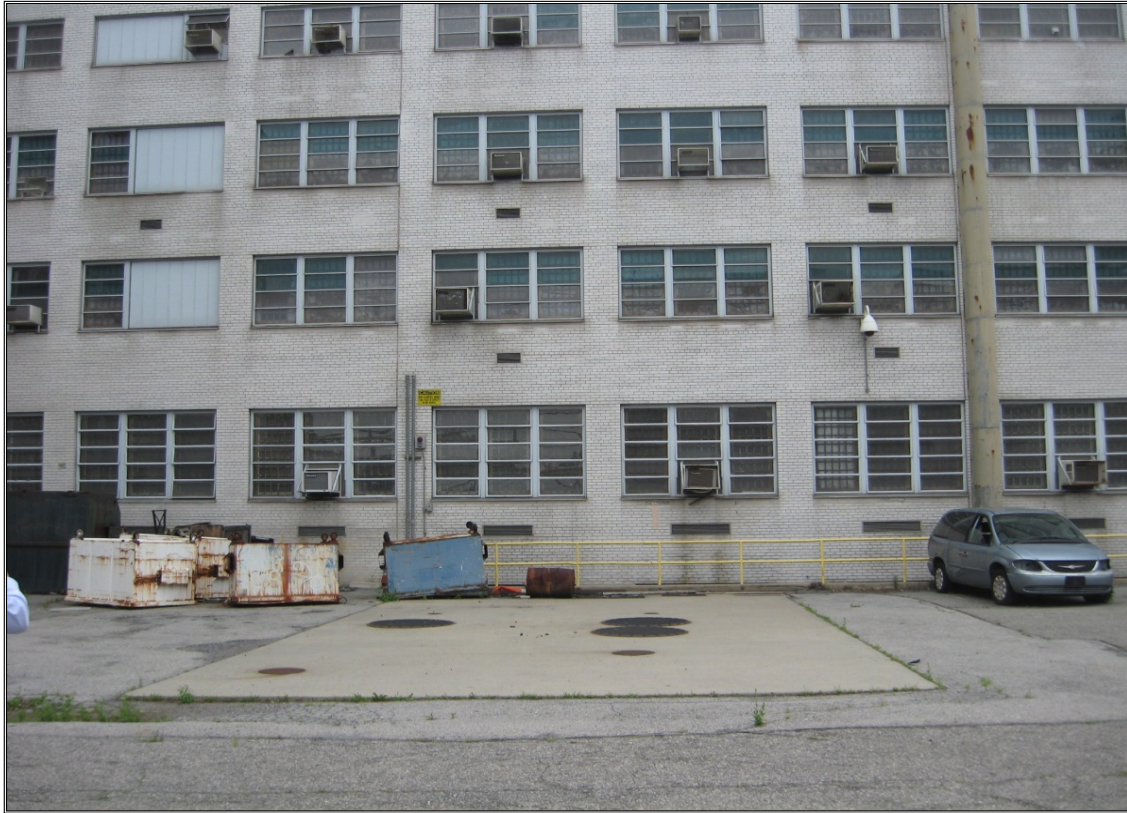
View north of UST area
