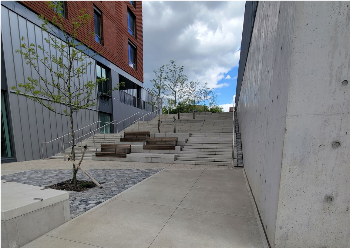
Photograph 3: Facing east, view of Site improvements in the courtyard area between Buildings 1A (left) and 1B (right).
