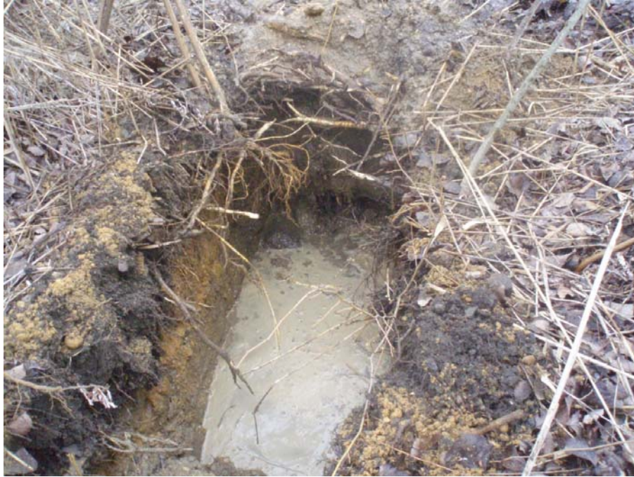
Photograph 3: Test Pit (along west edge of concrete slab)
