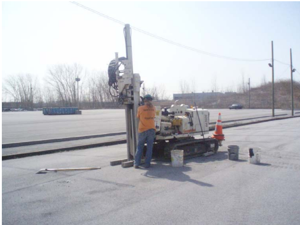
Photograph 4: Drilling Boring B18.
