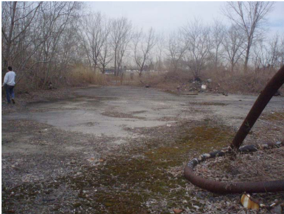
Photograph 2: Abandoned Concrete Foundation Slab
