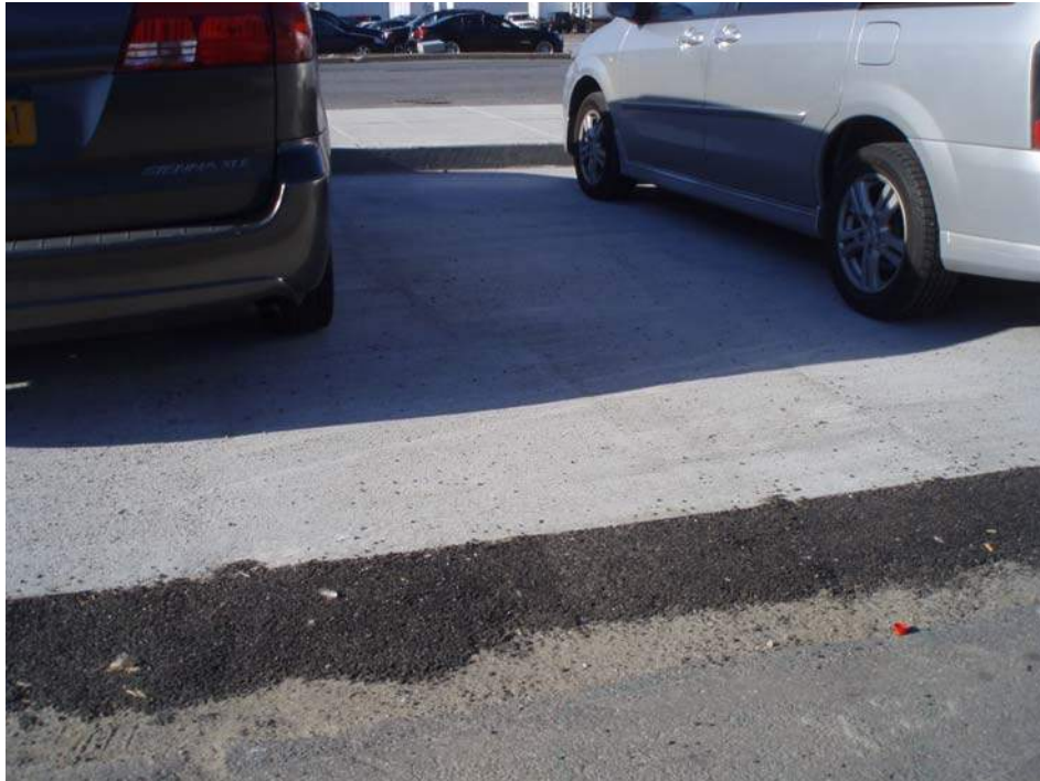
Photograph No. 5 – Asphalt patch along concrete installation.
